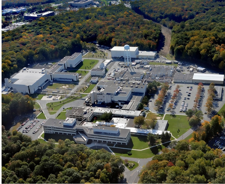
Exhibit 1-3. Aerial View of PPPL
