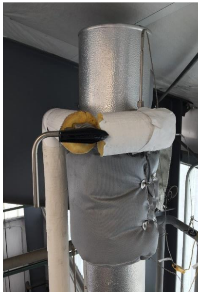
Figure 36: 3-way valve for online calibration of FT-300
