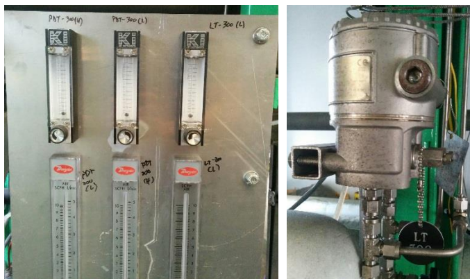
Figure 38. Flow control panel for N 2 purge taps (Left) and example of N 2 purge tap installation on one of the pressure transmitter (Right). N 2 enters through the horizontal tube at the tee.
