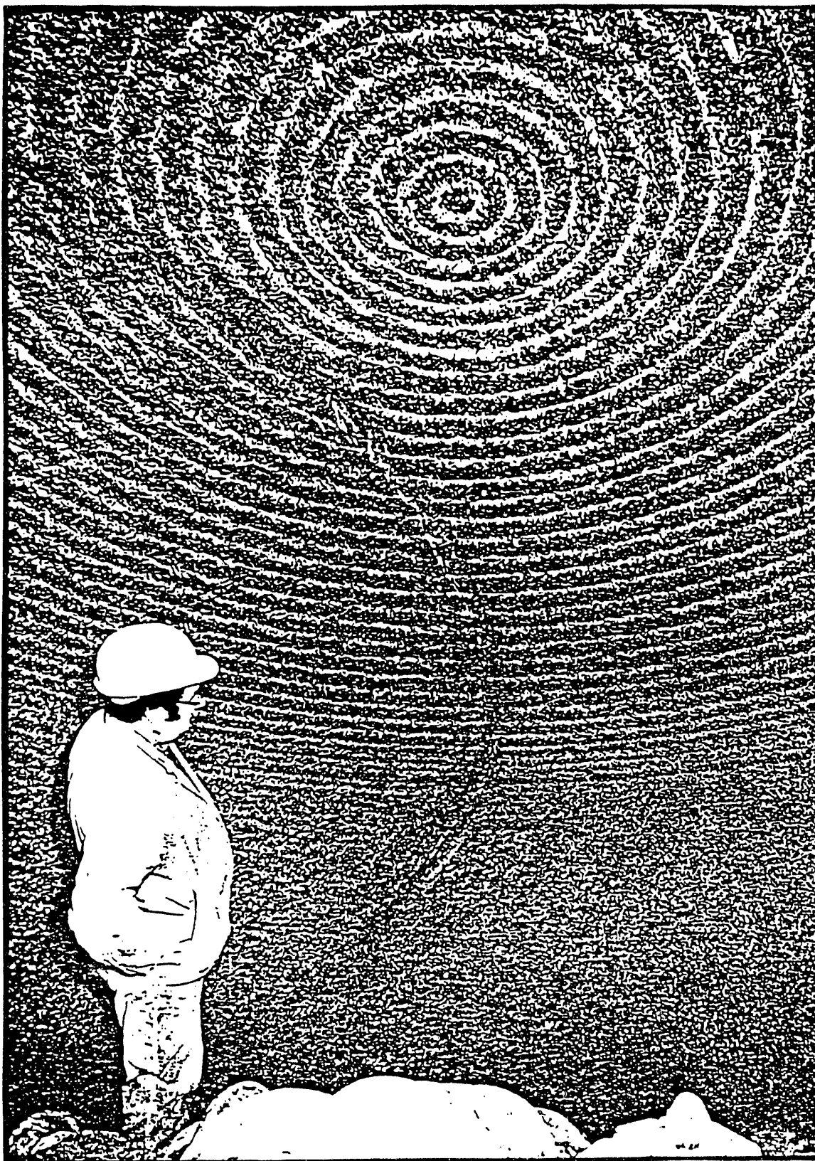
Figure 5. The Rock Face Left by a TBM. Note the circular cutter paths and the planar geologic feature on which the observer is standing.
