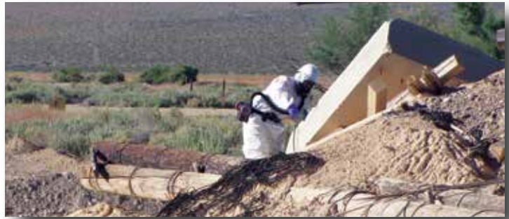
Radiological Control Technician performing a radiological survey of concrete debris at a Soils CAS on the NNSS in 2016.
