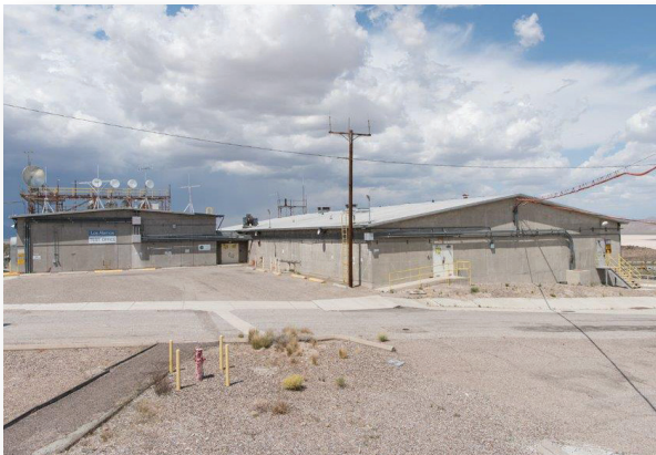
Control Point-1 (CP-1) Building
