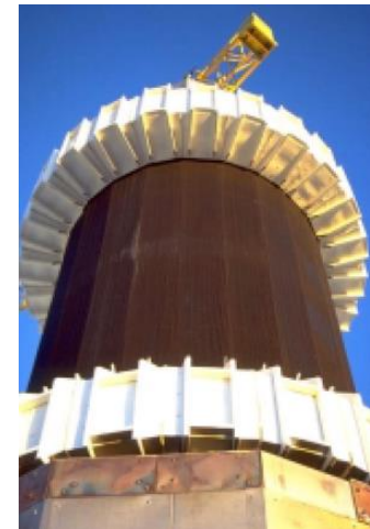
External tubular receiver
