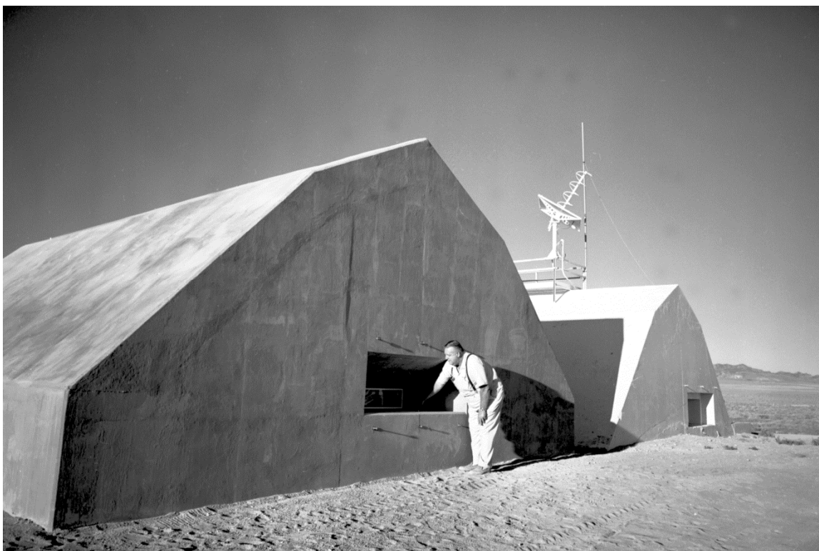
Figure 8 Unknown photographer. 1964. FIRE CONTROL BUNKER (BUILDING 09-51); WEST AND SOUTH SIDES; RECESSED OBSERVATION WINDOW; NEWLY COMPLETED BUILDING; CONCRETE STILL APPEARS DAMP; VIEW FROM SOUTHWEST
