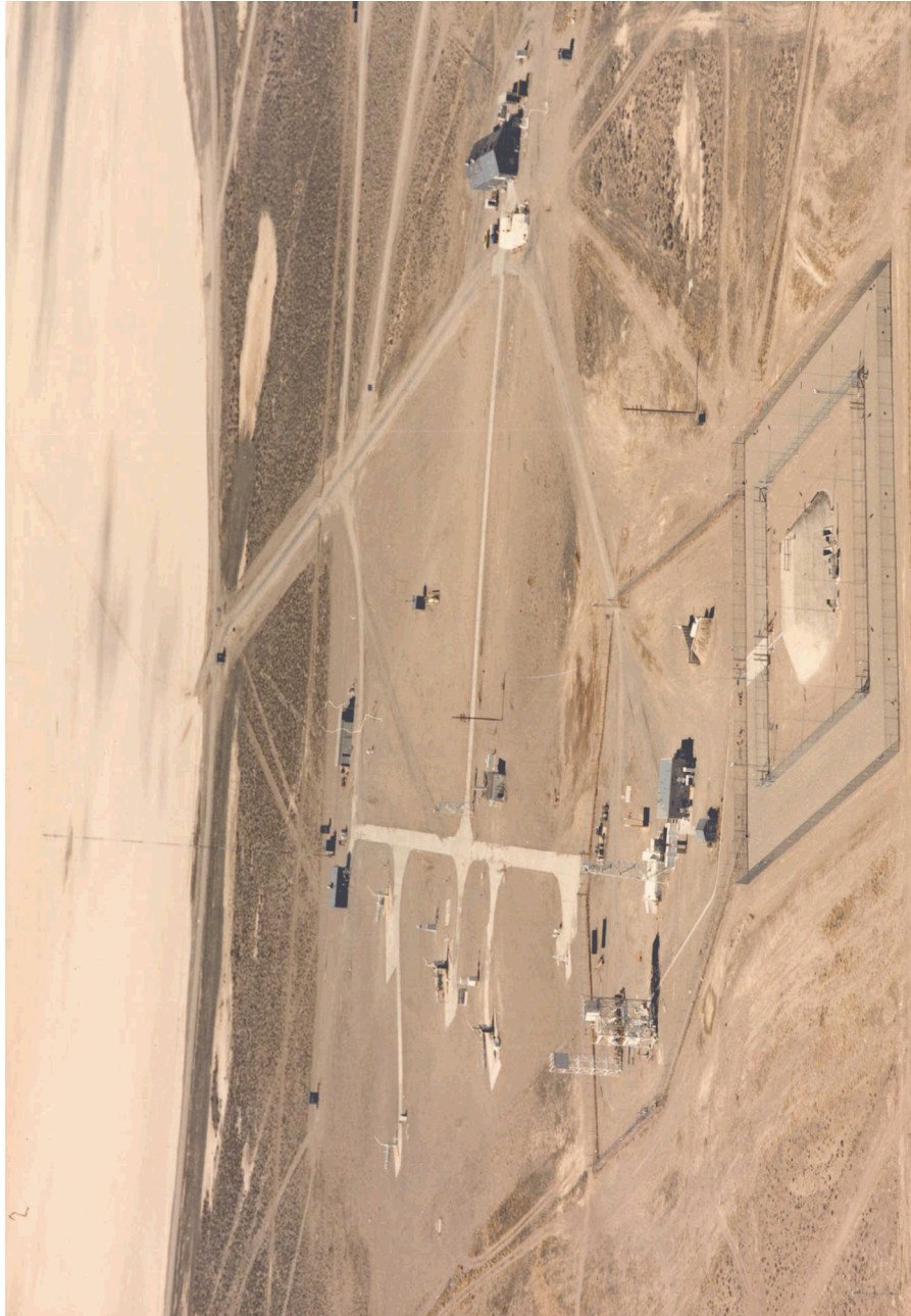
Figure 6 Photographer unknown. 1985. AREA 9, TONOPAH TEST RANGE; AERIAL PHOTOGRAPH; BUILDING 09-54 IS LEFT OF CENTER, IN FRONT OF BUILDING 80-00, 300' METEOROLOGICAL TOWER; VIEW FROM WEST
