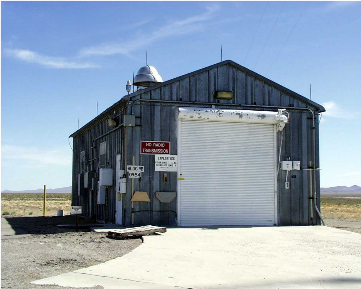
Figure 10 Clair Blackburn, Photographer. 2009. BUILDING 09-54, EXTERIOR; NORTH END OF BUILDING; ROLL- UP DOOR AND POURED CONCRETE DRIVEWAY; ASSEMBLY BUILDING 9B; VIEW FROM NORTHEAST
