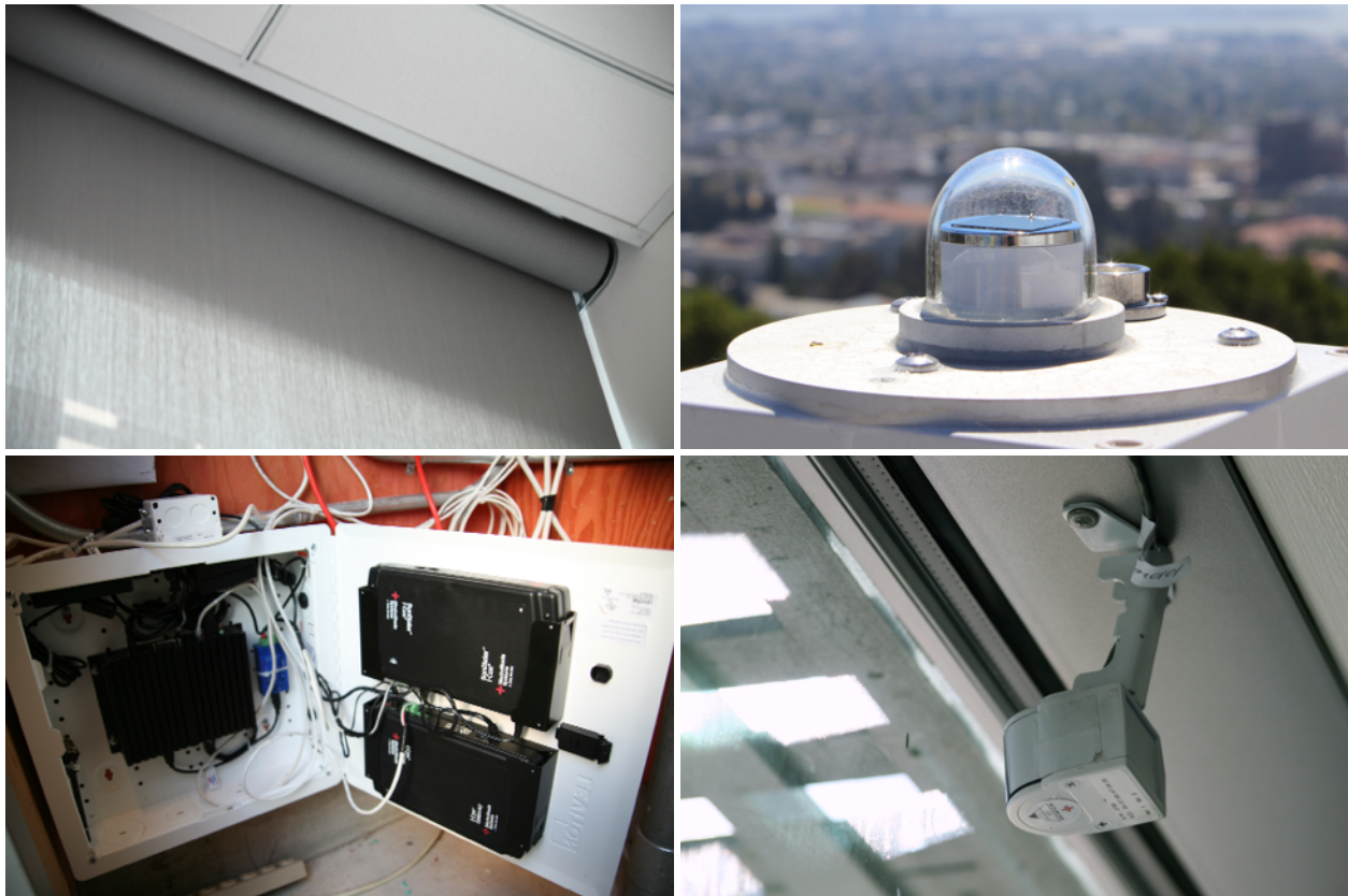
Figure 7.1 - Photographs of MechoSystems components. Clockwise from top left: motorized roller shade (medium grey color), rooftop irradiance sensor, illuminance sensor mounted to the window frame, MechoSystems control cabinet.
