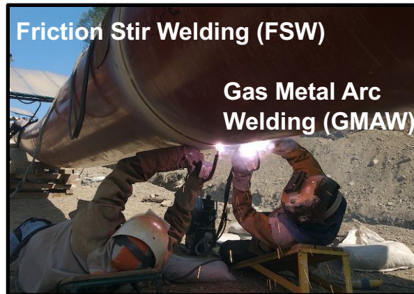
Welding to join or repair pipe
