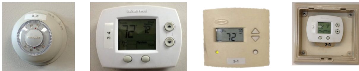
Figure 9-4. Sample pictures of existing thermostats before BEMOSS™ deployment
