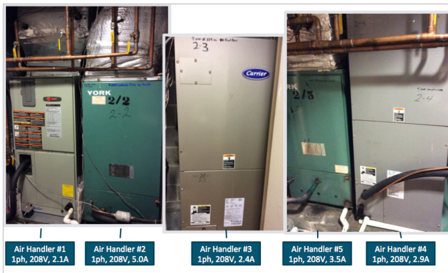
Figure 9-6. Air Handlers serving the second floor
