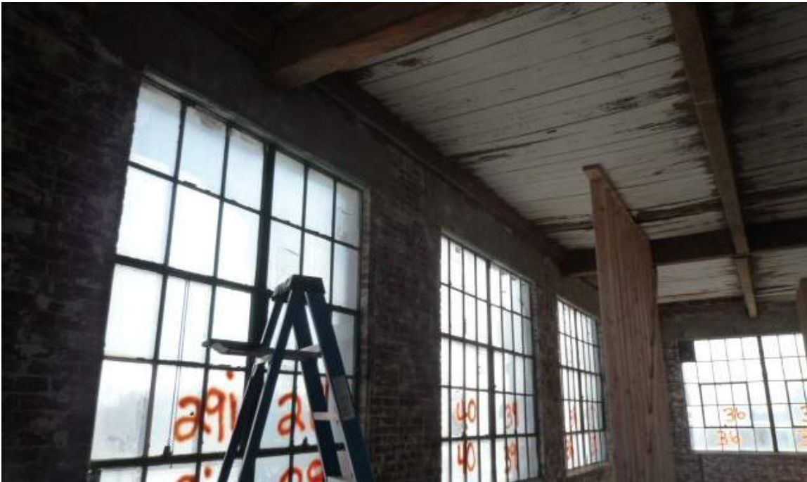
Existing ceiling, decking failure
