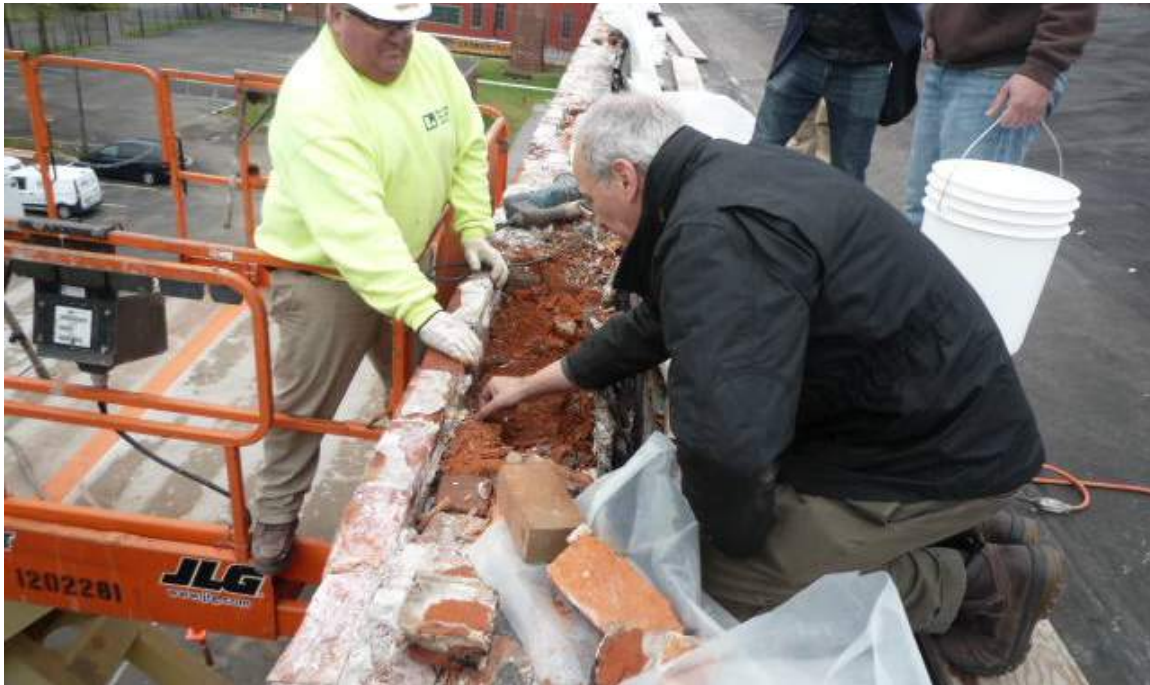
Engineer reviewing masonry deterioration
