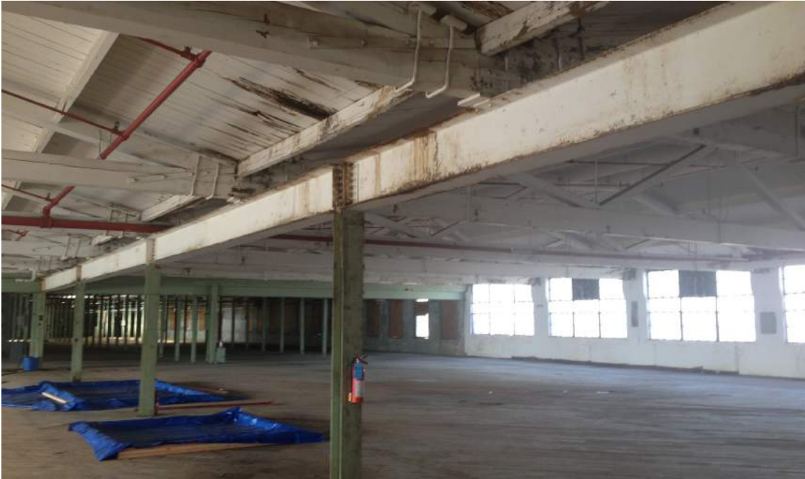
Existing truss and roof, leaking
