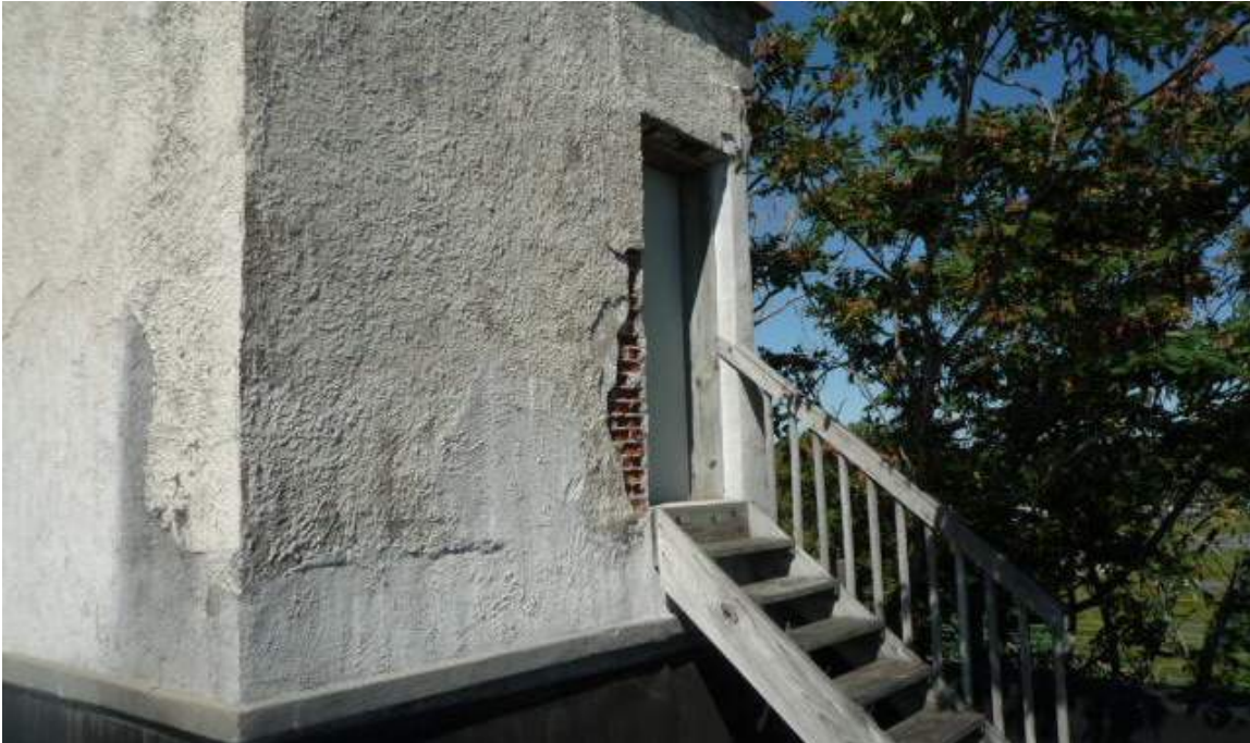
Existing elevator bulkhead, failing mat'l
