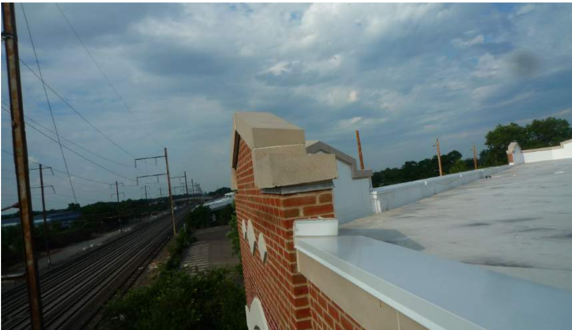
Rebuilt raised parapet
