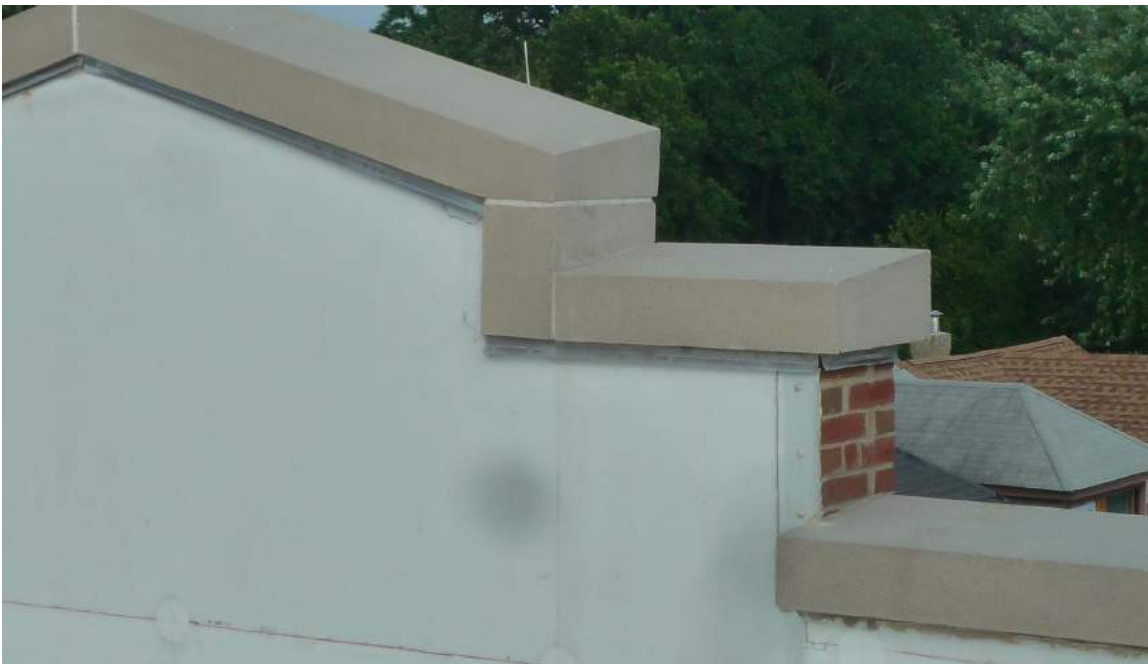
Rebuilt parapet and coping stones
