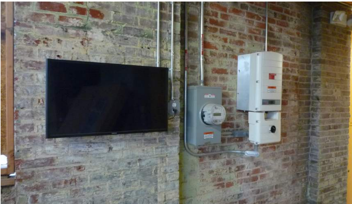
Solar meter and inverter, first floor hallway
