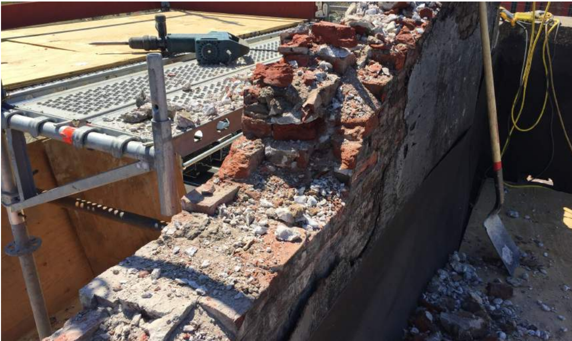
Demolishing deteriorated parapet
