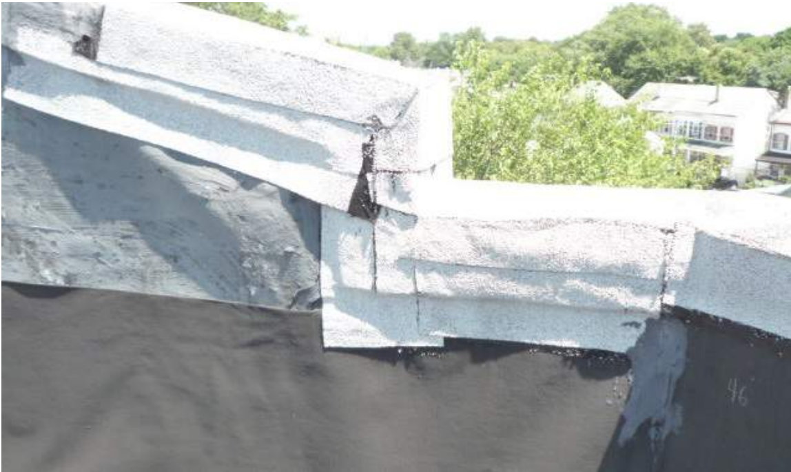
Coping at raised parapet
