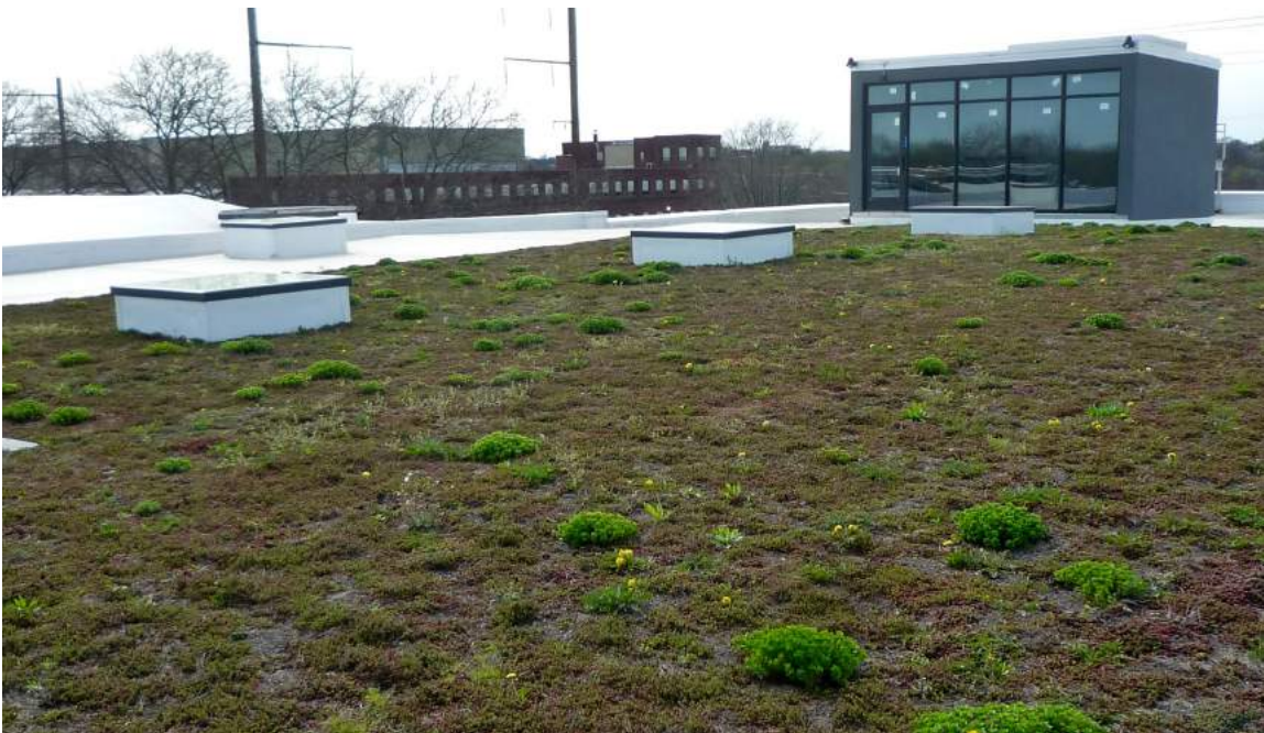
Green roof – retains 8,000 gallons of water in heavy rain
