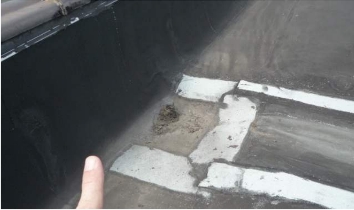
Existing 3 built up layers of roof
