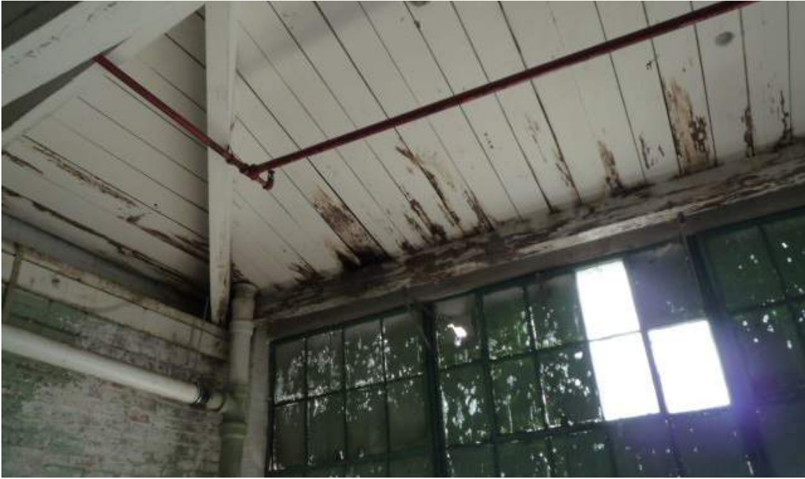
Existing ceiling, rot at low points
