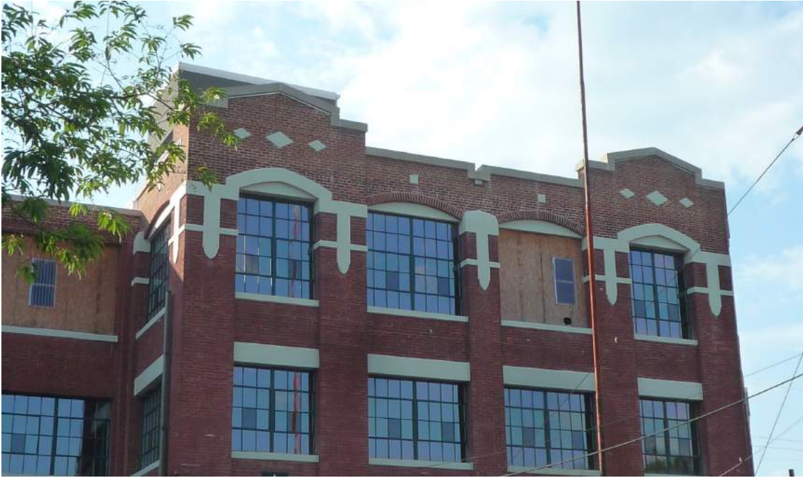
South façade – parapet rebuild, medallion replacement
