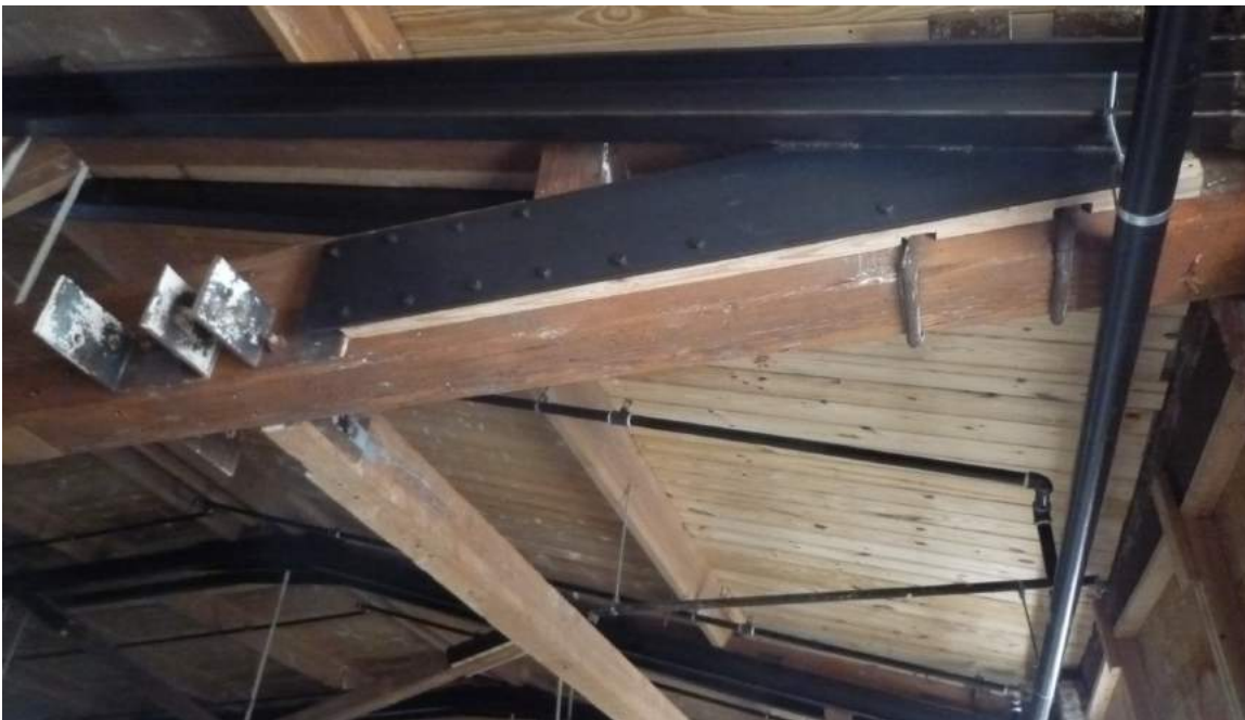
Truss reinforced, decking replaced
