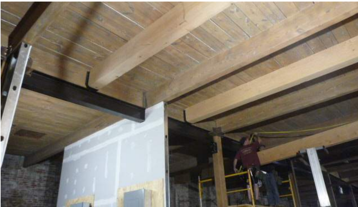
New decking and structural reinforcement
