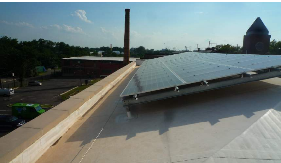
Rebuilt parapet and solar PV panels
