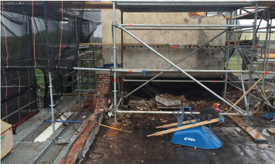
All parapets and elevator bulkhead rebuilt from roof up
