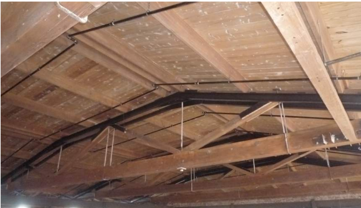
Trusses cleaned and reinforced, future event space
