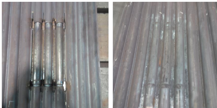
Figure 3-m Shop Repair of T92 Panel Before Fill Out and After PWHT
