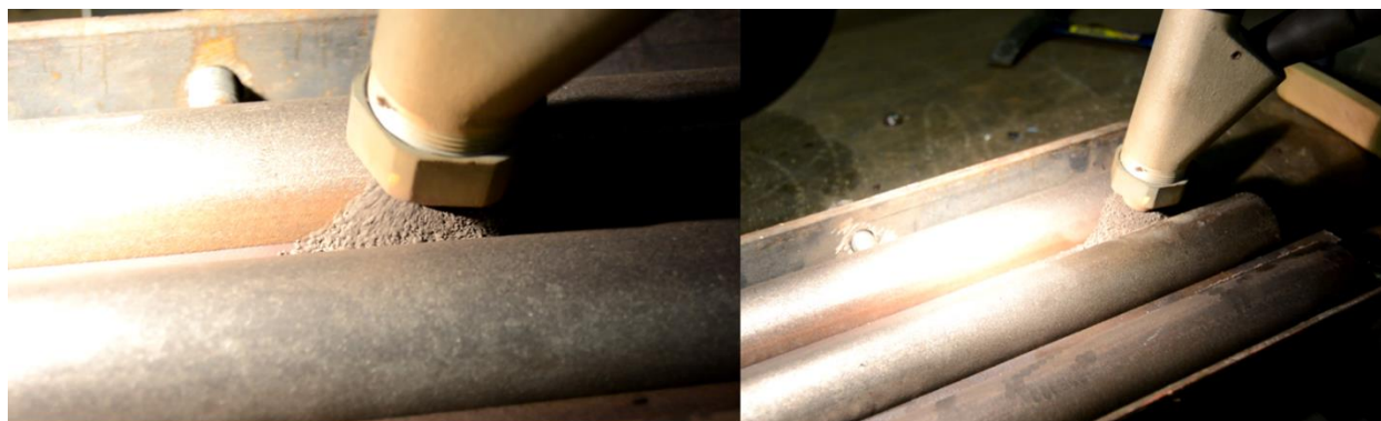
Figure 3-b Welding of T92 Panel with Sub Arc Process
