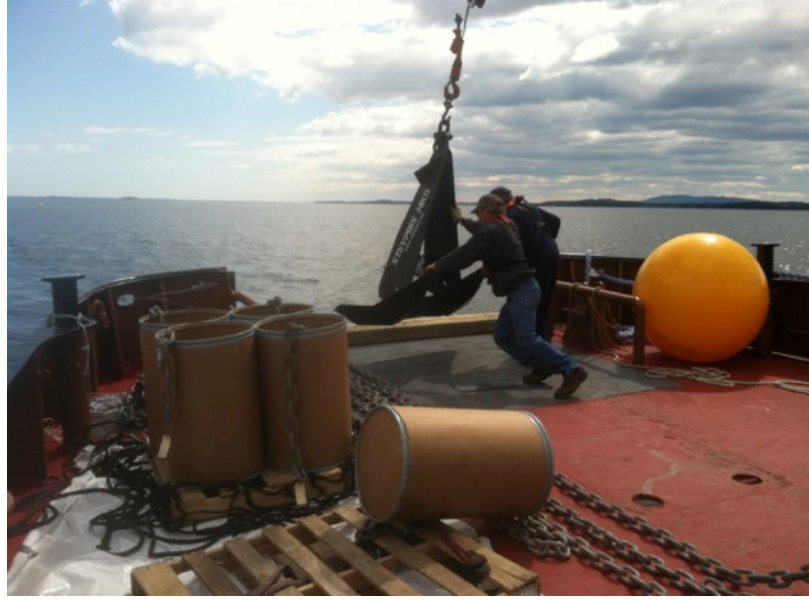
Figure 24 Drag Anchors being lowered into water
