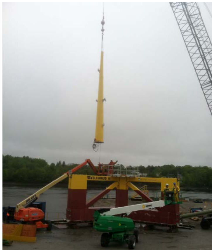
Figure 20 Installation of Tower at Cianbro Facility in Brewer
