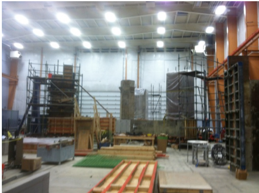
Figure 16 Bottom Beams Cast, Radial Columns Poured
