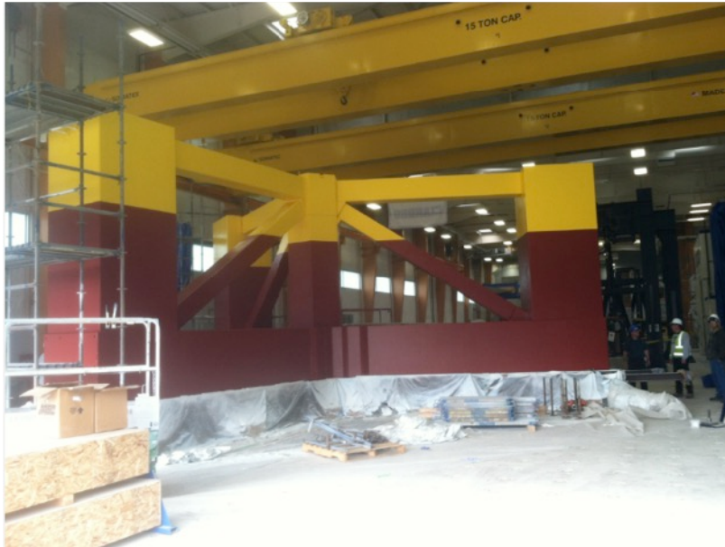
Figure 19 Top Beams Inserted and Painting Complete
