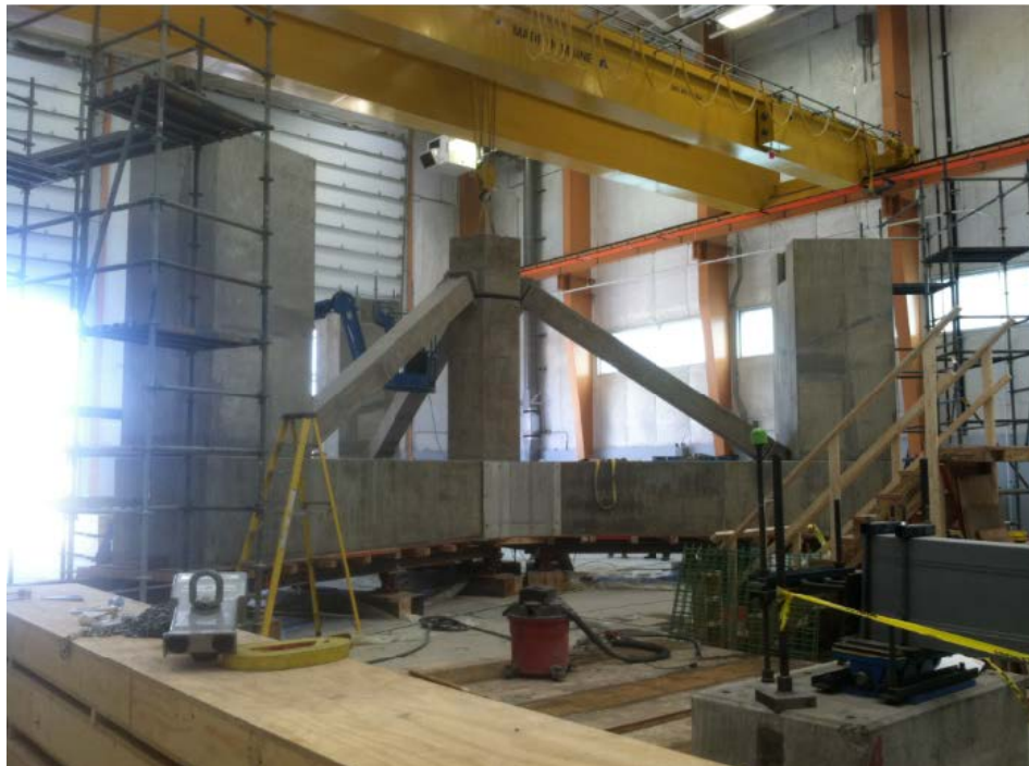
Figure 18 Compression Struts Installed
