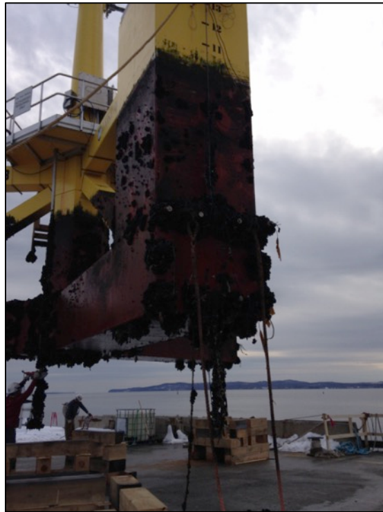
Figure 39 Marine Growth on the VoltturnUS 1:8 Hull
