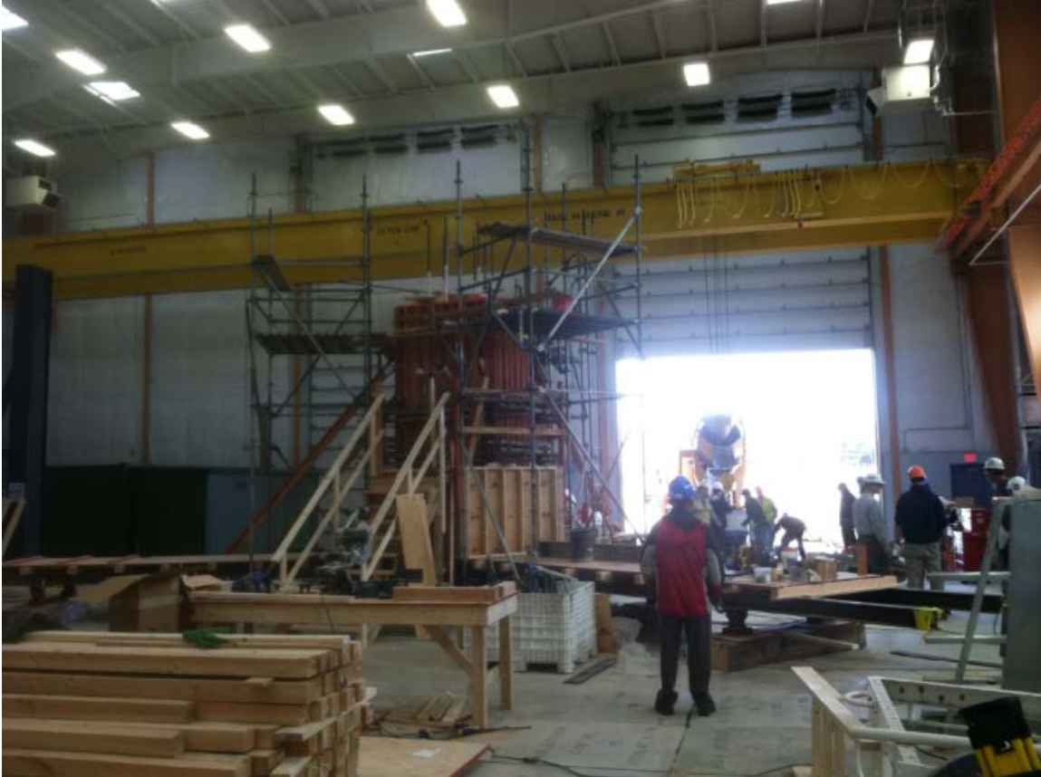
Figure 14 Concrete Formwork for VoltturnUS Center Column and Bottom Beam Slabs
