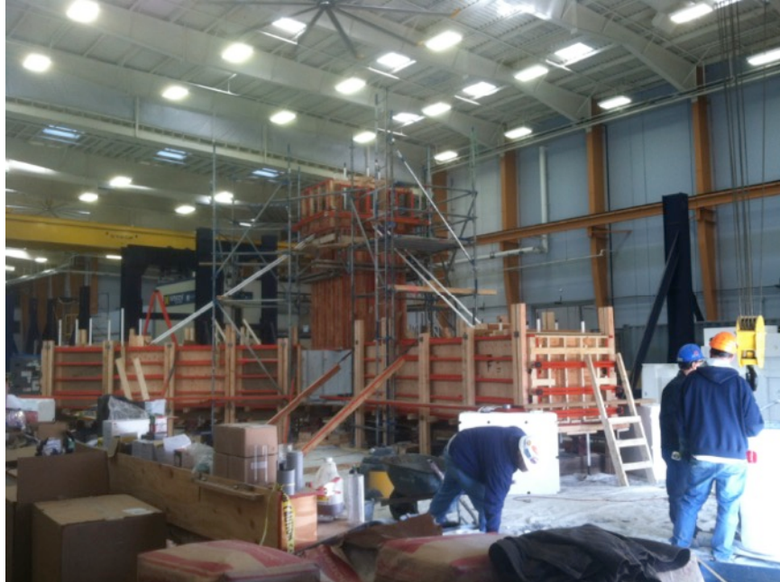
Figure 15 Bottom Beams Form Work in Place
