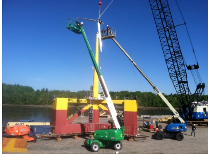
Figure 21 Installation of Turbine
