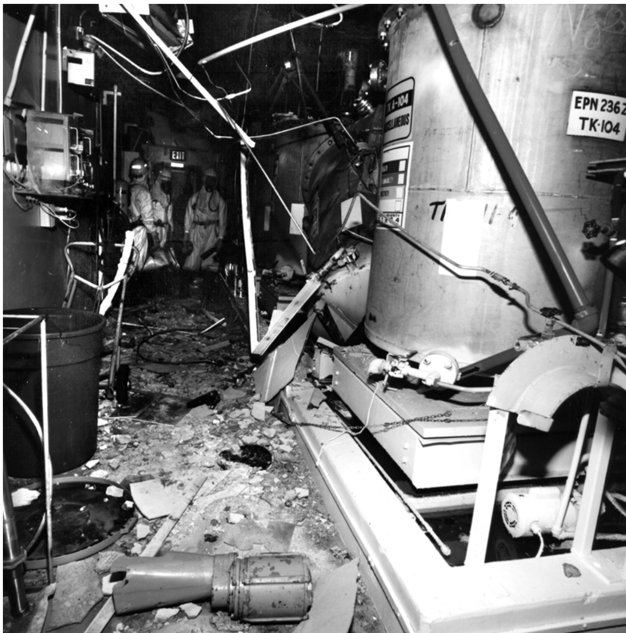
PRF Accident Scene in the Plutonium Finishing Plant, May 14, 1997
