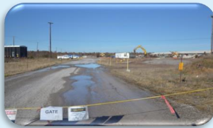
C-746-B warehouse after.
