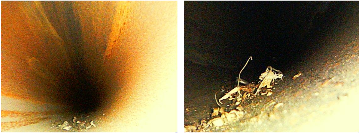
Figure 13: Figure 40. Images of debris within the expansion tanks, as captured by borescope.
