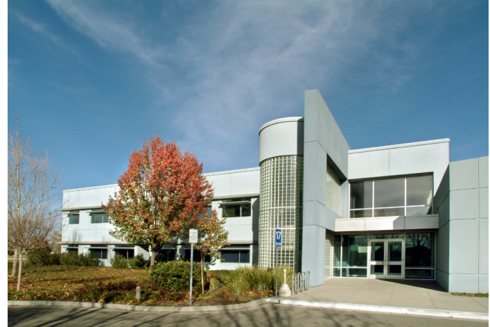
LLNL's National Atmospheric Release Advisory Center facility includes an operations room, a dedicated computer center, redundant communications systems, and 24/7 electrical power systems.
