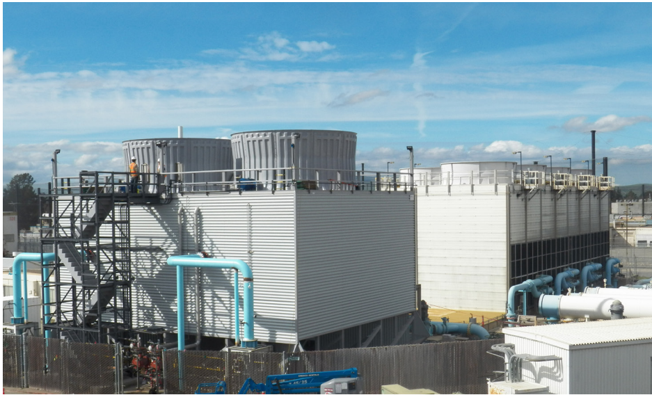
Cooling towers at the Central Utility Station (U235) were recently replaced, which revitalized a critical part of the site-wide low-conductivity water system.
