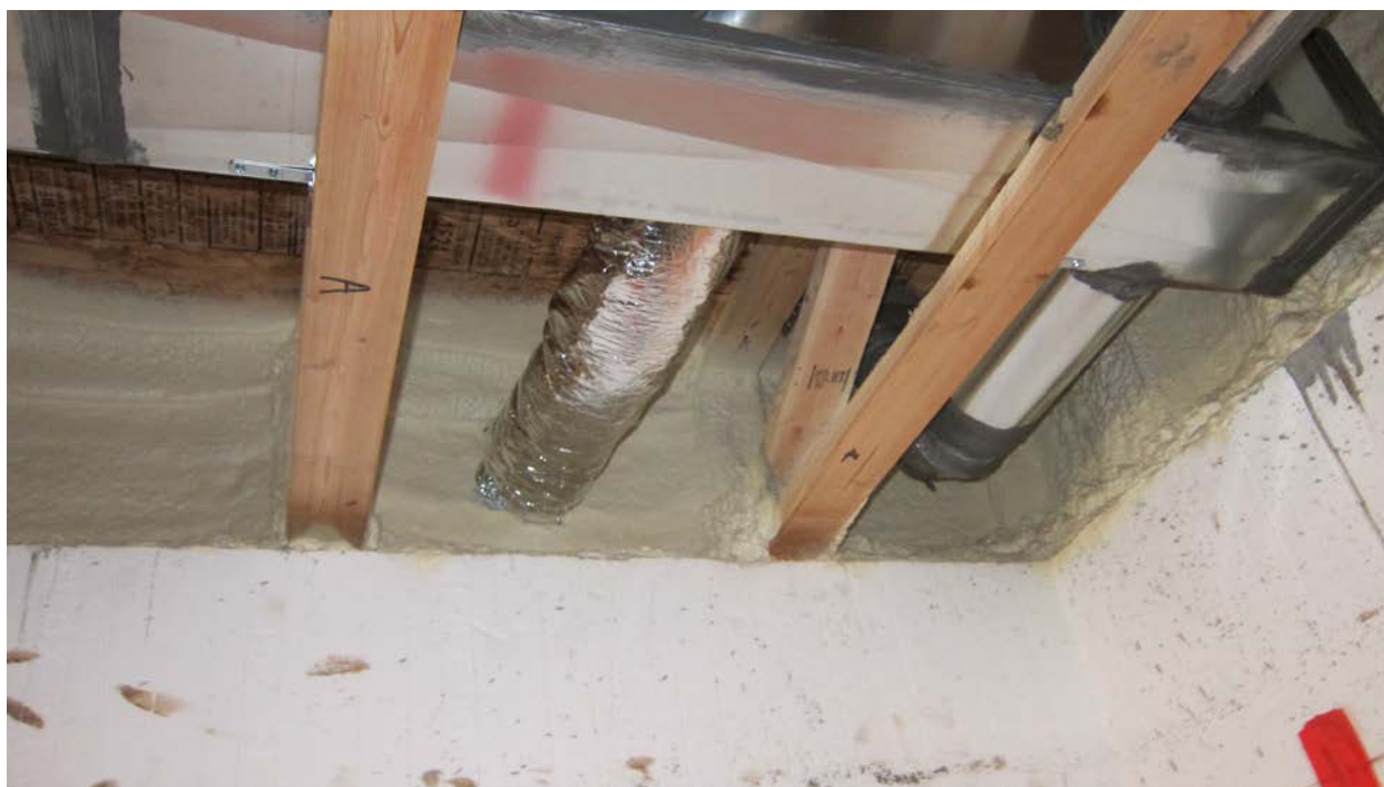
Figure 32. Urban Homeworks: ICF foundation, closed-cell spray foam at rim joist, and sealed ductwork located within the thermal enclosure of the North Minneapolis, Minnesota, project
