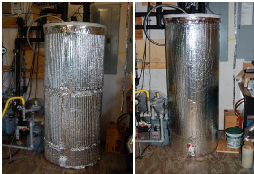
Figure 16. Argon gas-filled wrap (left), triple-layer bubble wrap (right)
