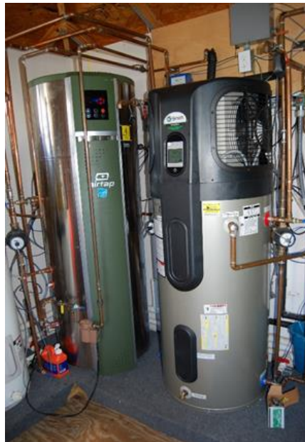
Figure 3. Two heat pump water heaters of large and medium storage capacity (80 and 60 gallons)
