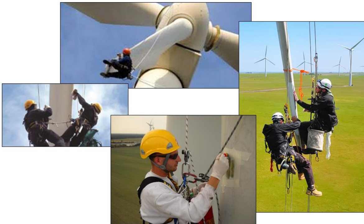
Figure 2-13: Use of Skyworkers to Access Blades Via Climbing Ropes
