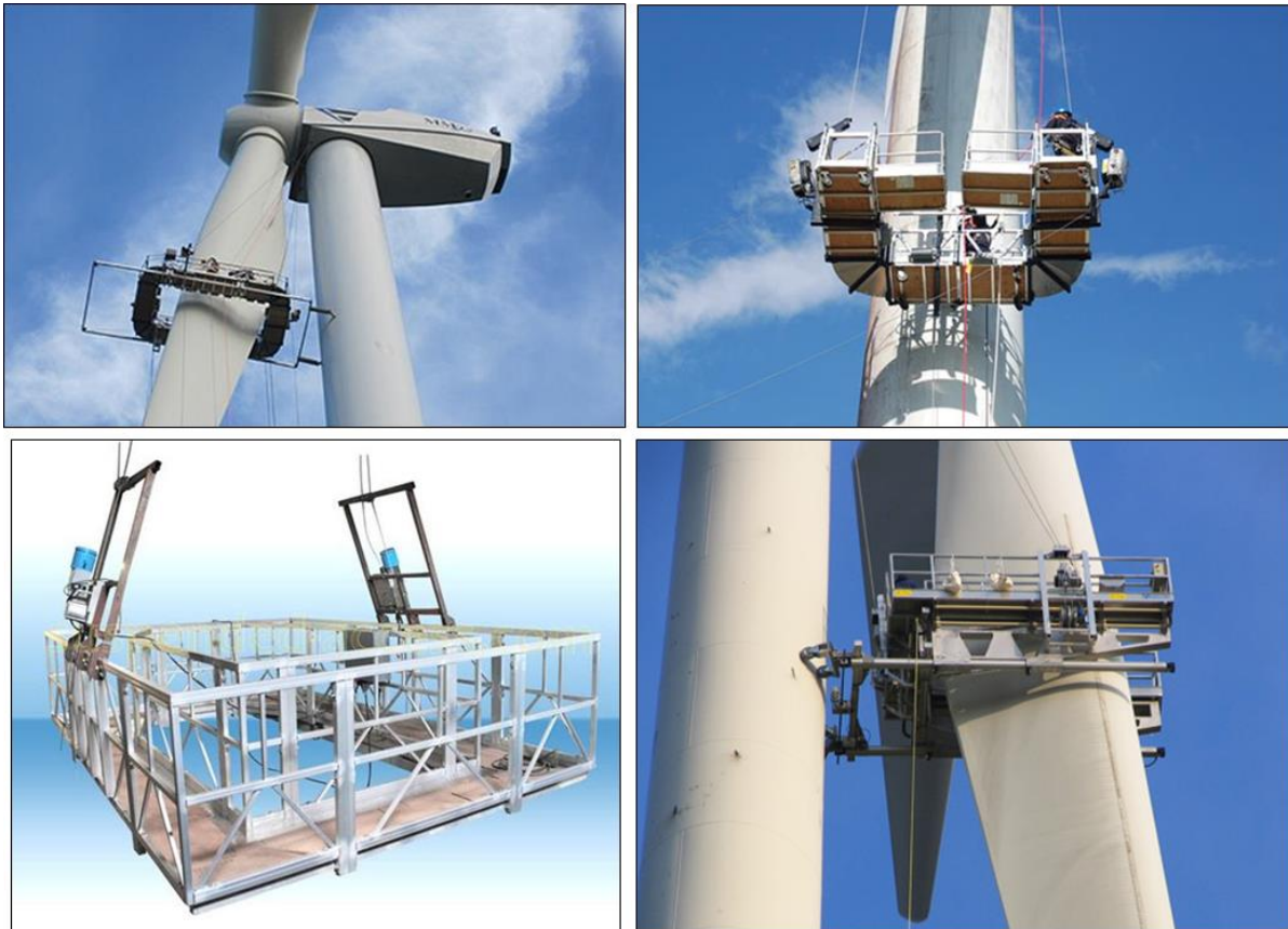
Figure 2-14: Use of Adaptive Platforms to Provide Larger Work Space for Blade Maintenance Activities
