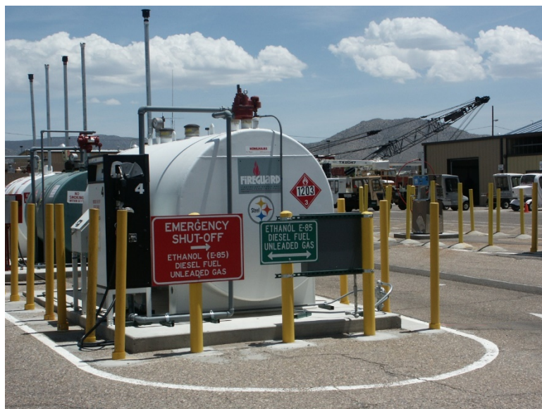
Aboveground storage tank
