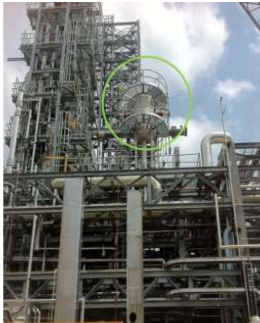
Figure 29. CSTR – PSTU Integration: CSTR Installed at NCCC (Q3 2015)
