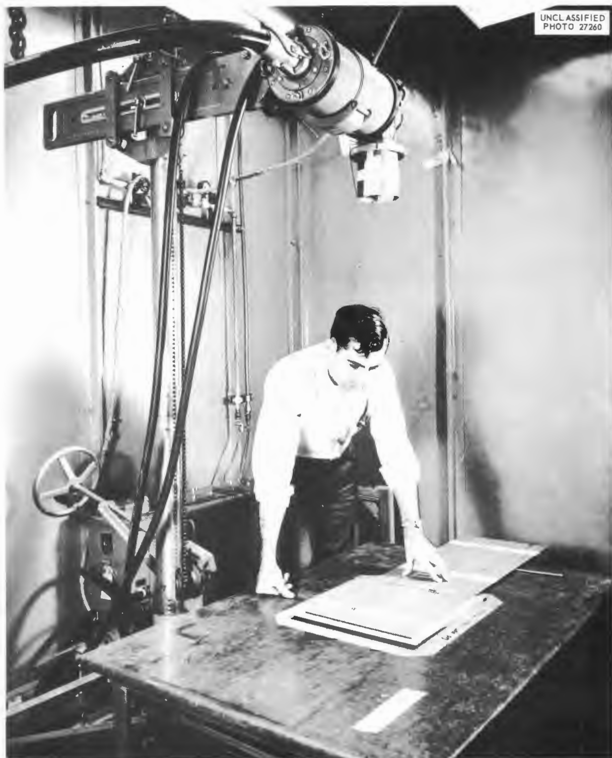
Fig. 3.7.4. Group of Tubes in Position for Radiography.
