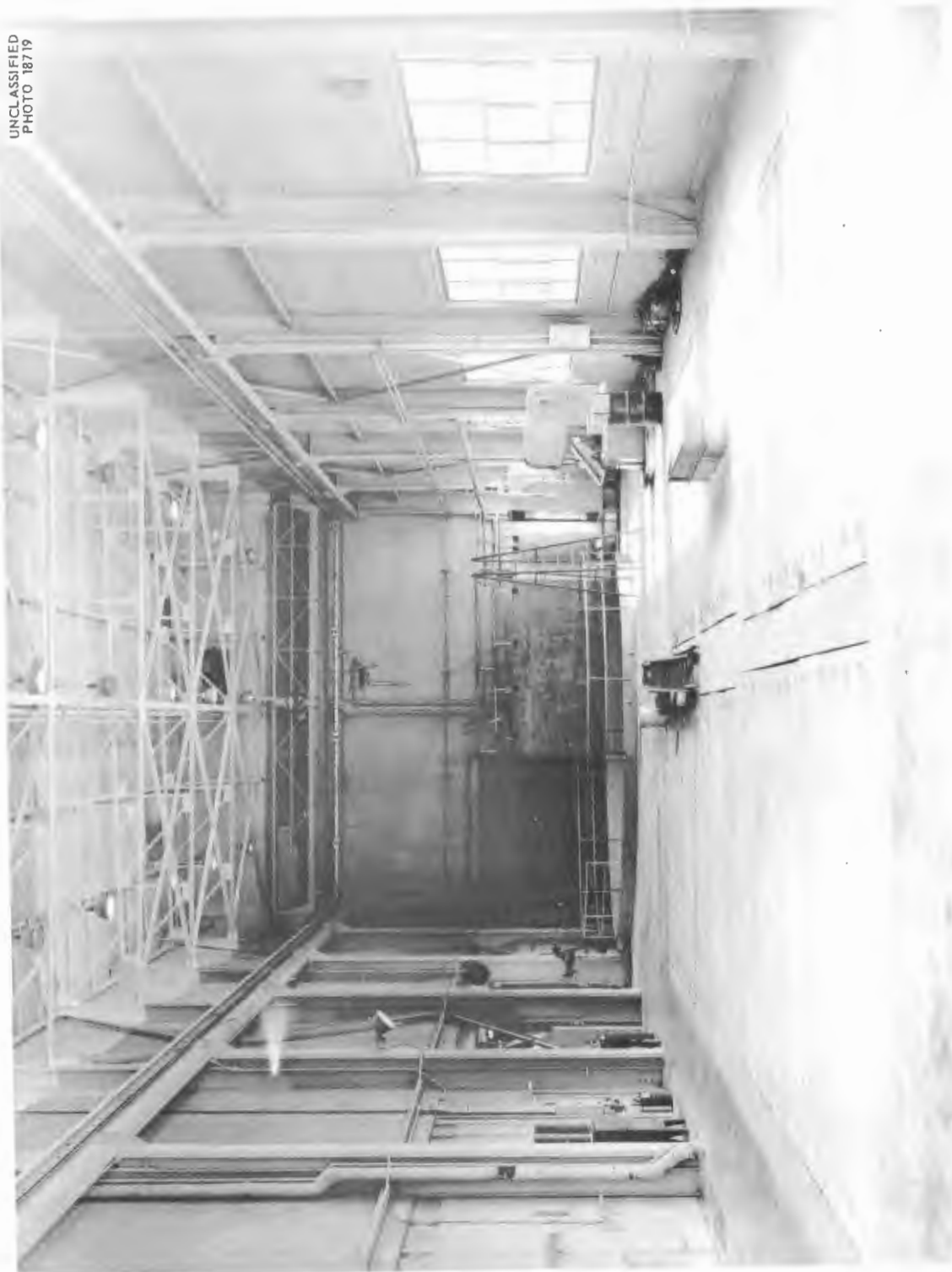
Fig. 1.5.3. ART Facility Crane Bay After Removal of Parapet Walls on ARE Pits.
