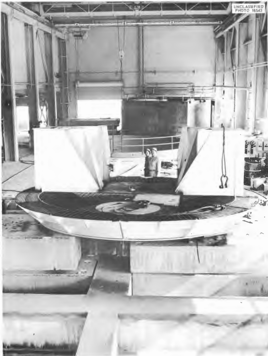
Fig. 1.5.1. Floor Structure Ready for Installation in Cell.
