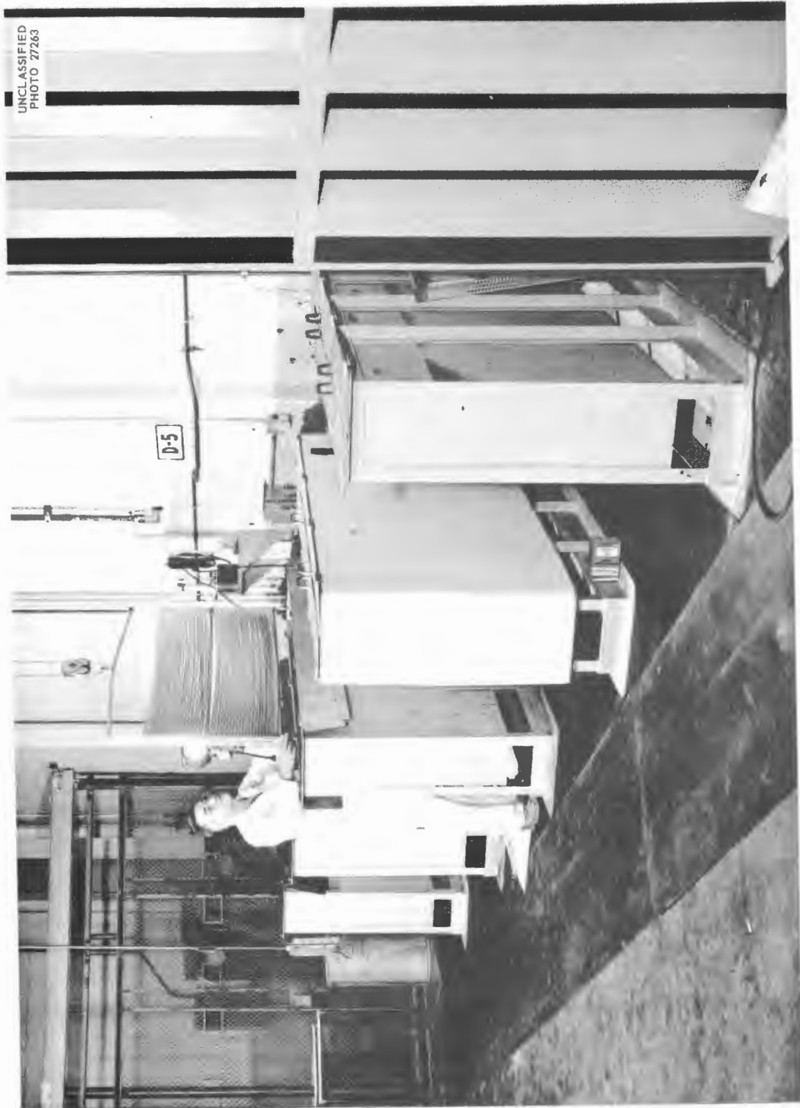
Fig. 3.7.2. Equipment for Fluorescent-Penetrant Inspection of Tubing.
