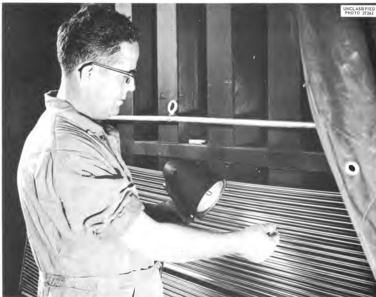
Fig. 3.7.3. Inspector Examining Tubing for Fluorescent-Penetrant Indications.
