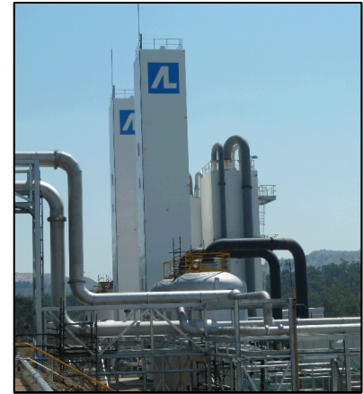
Dual cryogenic separation towers, Callide Oxyfuel Demo Project, Australia
