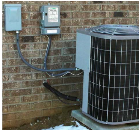
Figure 5. Schematic of direct load controller switching system. Source: Oregon PUC
