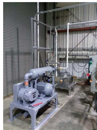
Exhibit 10. Picture of permeate blower installed at 0.1 MWe bench scale skid
