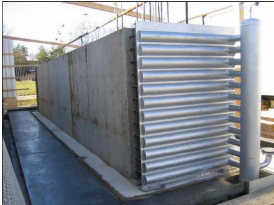
Figure 29. Example of a concrete thermal energy storage module [110].
