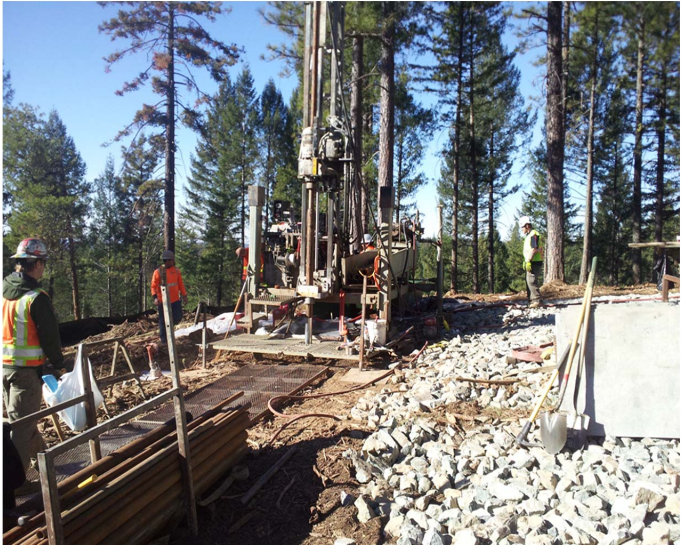
Figure 2. Core Hole Drilling at CH-3 within the proposed upper reservoir footprint of the Iowa Hill Pumped-storage Project.
