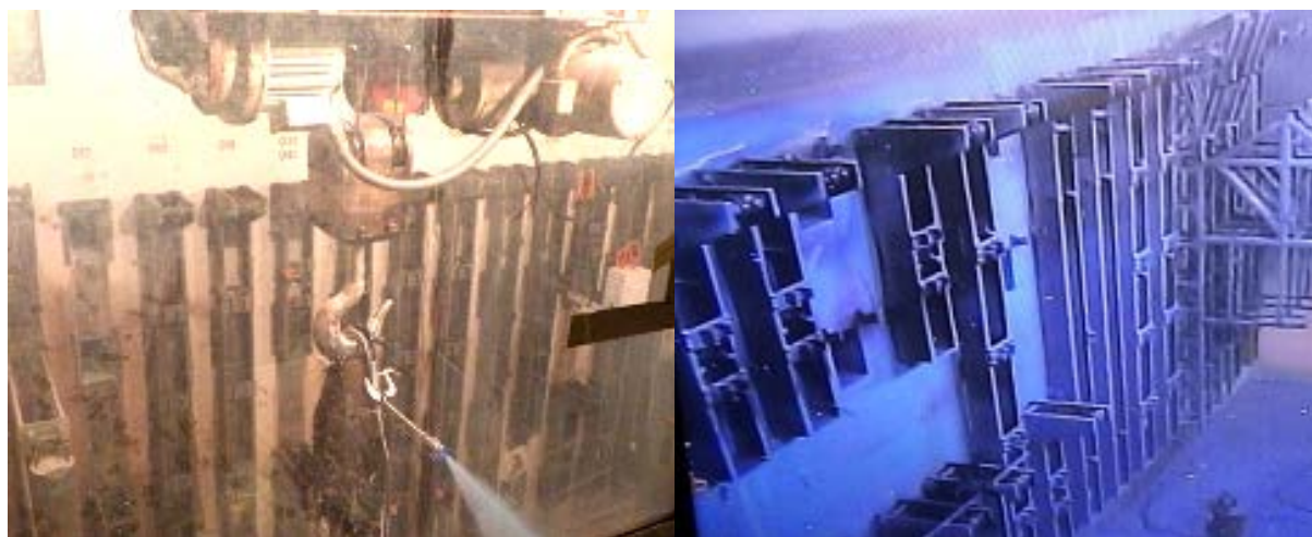
Fig. 1, Spraying PBS at the PFP/PRF and “Fixed” Contamination in Blue.
