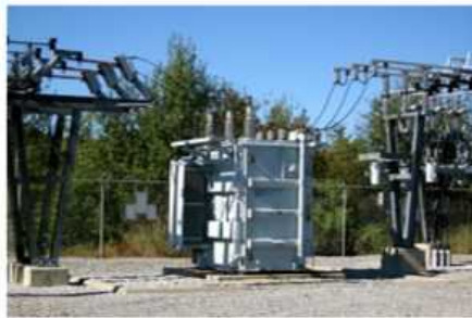
8000 lbs, 60 Hz Distribution Transformer
