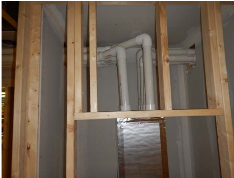
Figure 27. Final connections at plenum manifold
