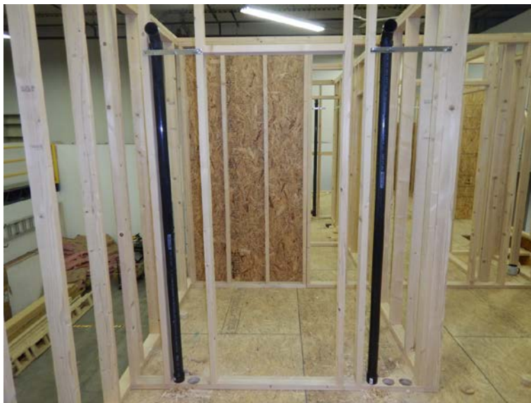
Figure 29. High-sidewall outlets
