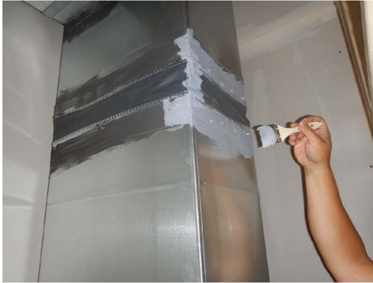
Figure 20. Plenum sealing
