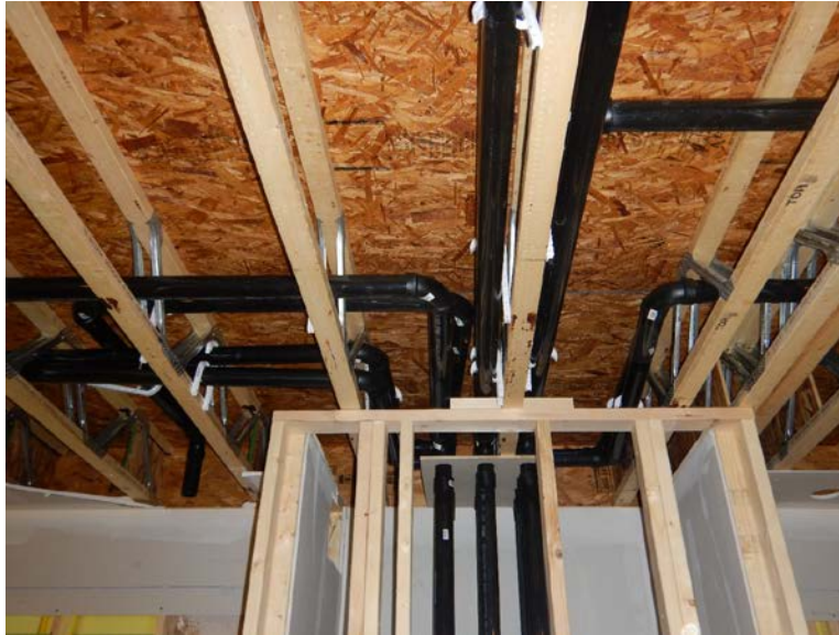
Figure 33. Pipe distribution through floor
