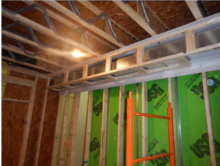
Figure 22. Framed ceiling chase
