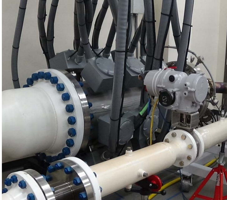
Figure 3-16. Primary Heater after Installation
