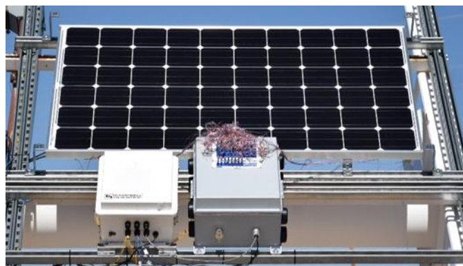
Fig. 1. 60 cell module mounted on tracker with data loggers
