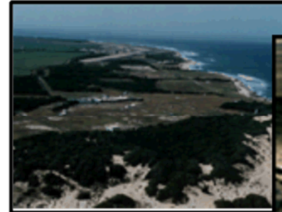
Kauai Test Facility Hawaii
