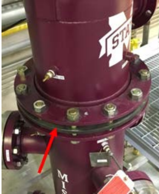
Figure 4.15 Tube sheet installed between housing section and housing cap.
