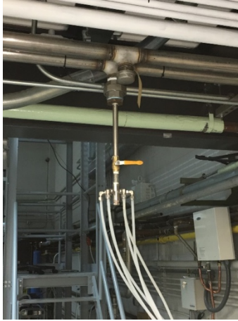
Figure 7.2 Tubing assembly to connect water line to filter elements.
