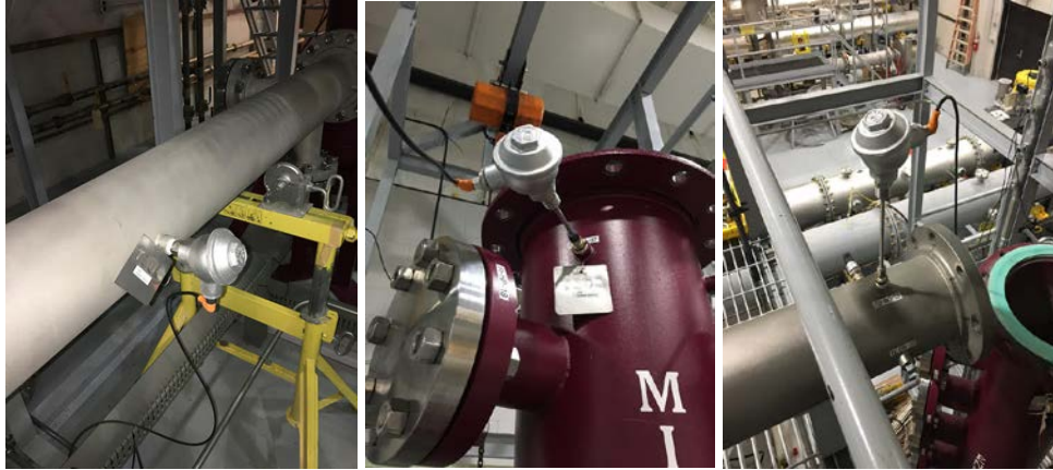
Figure 4.11 High temperature thermocouple and transmitter assembly.
