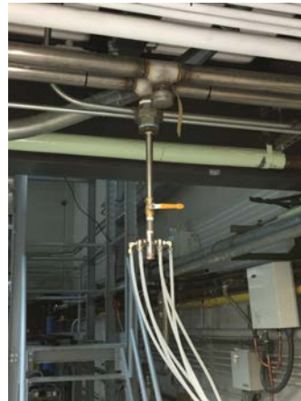
Figure 2. Tubing connecting the Type II water line to the filter elements.
