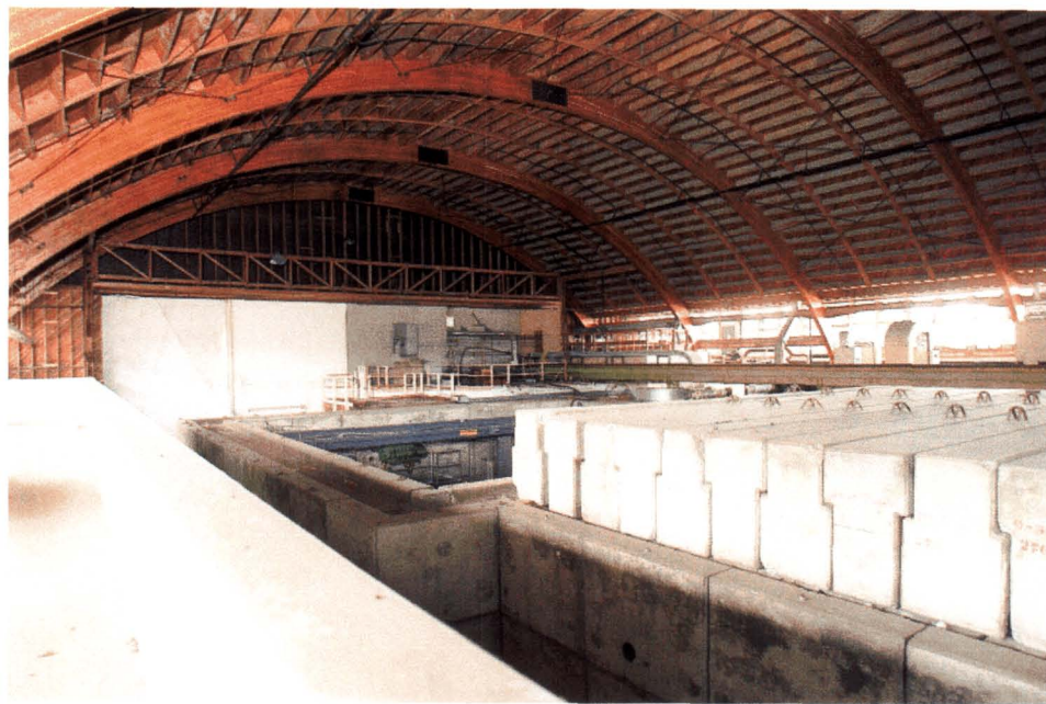
Figure 171. Freestanding wood laminated arches, Building 212, 2003. 742
