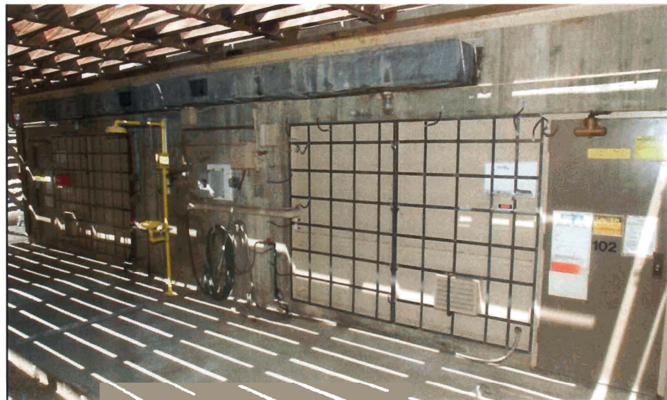
Figure 136. Building 825, frangible exterior walls, west elevation, 2003. 664
