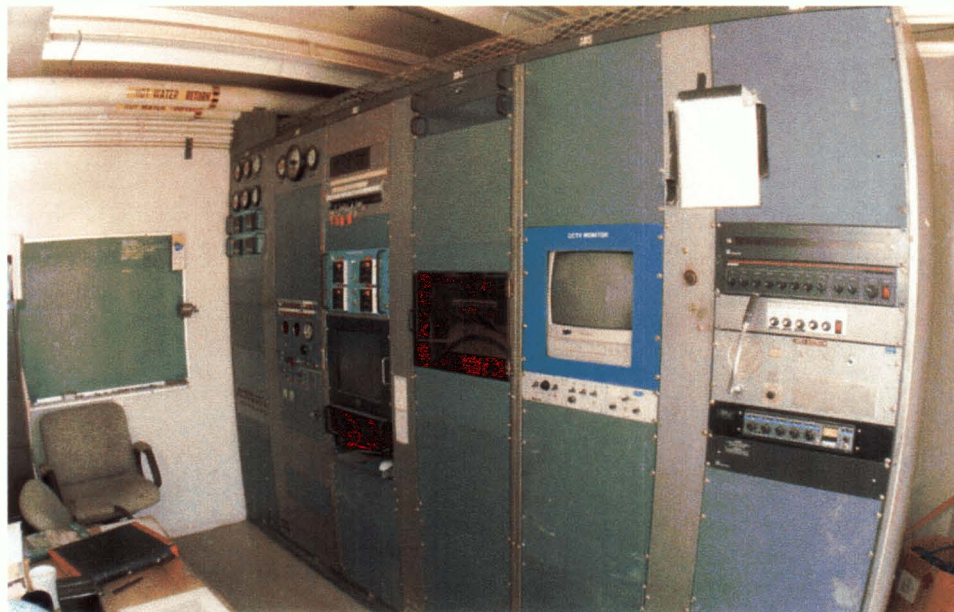
Figure 132. Control panel for remote-controlled ovens and presses, Building 817A, 2003. 652
