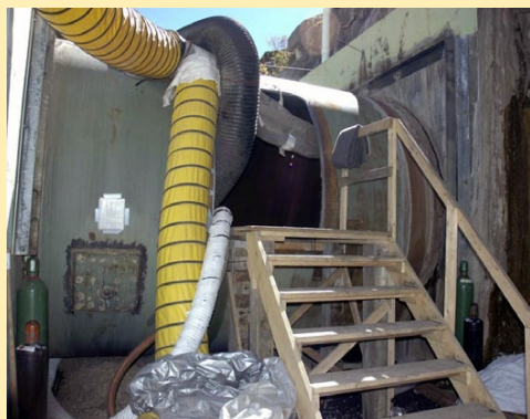
Figure 3. Access door cut into the penstock for recoating work.
