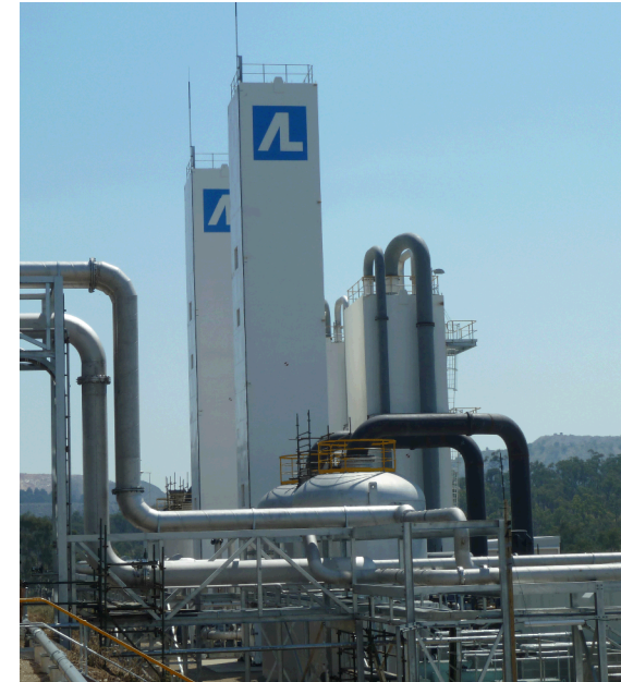
Air Liquide cryogenic ASU at Callide 30 MW e Oxy-Fuel Power Plant Demonstration
