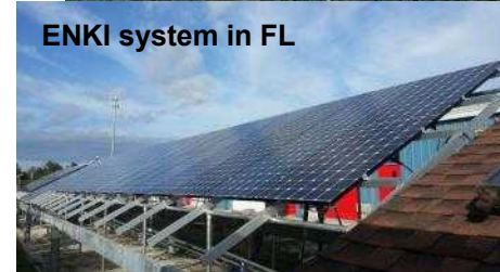
Maxim racks and combiners ready for modules in Florida
