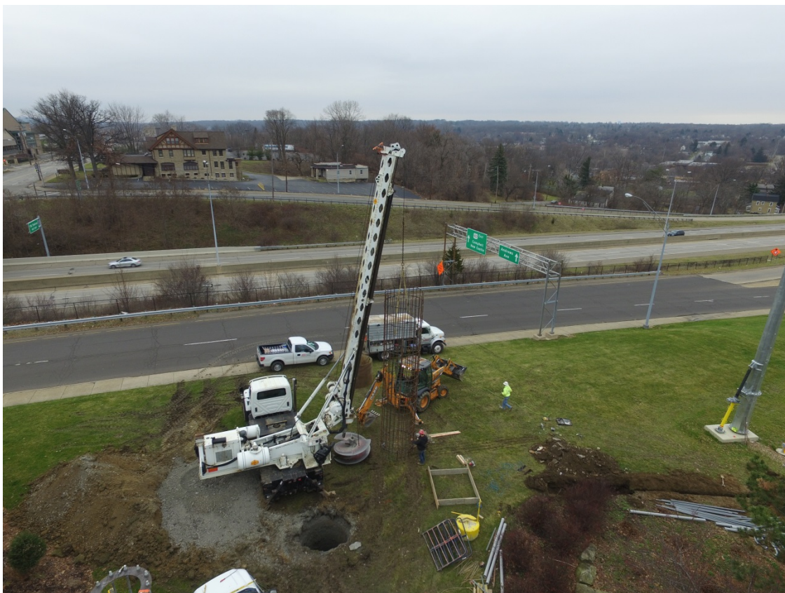
Figure 53. Foundation Preparation for Shrouded Wind Turbine
