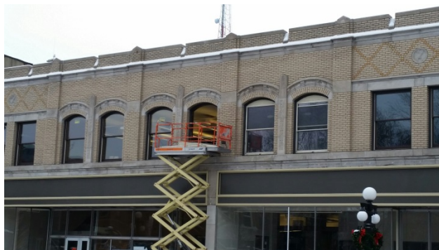
(a) Installation of new arch-top front windows
