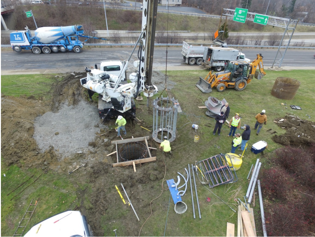
Figure 54. Foundation Preparation for Shrouded Wind Turbine
