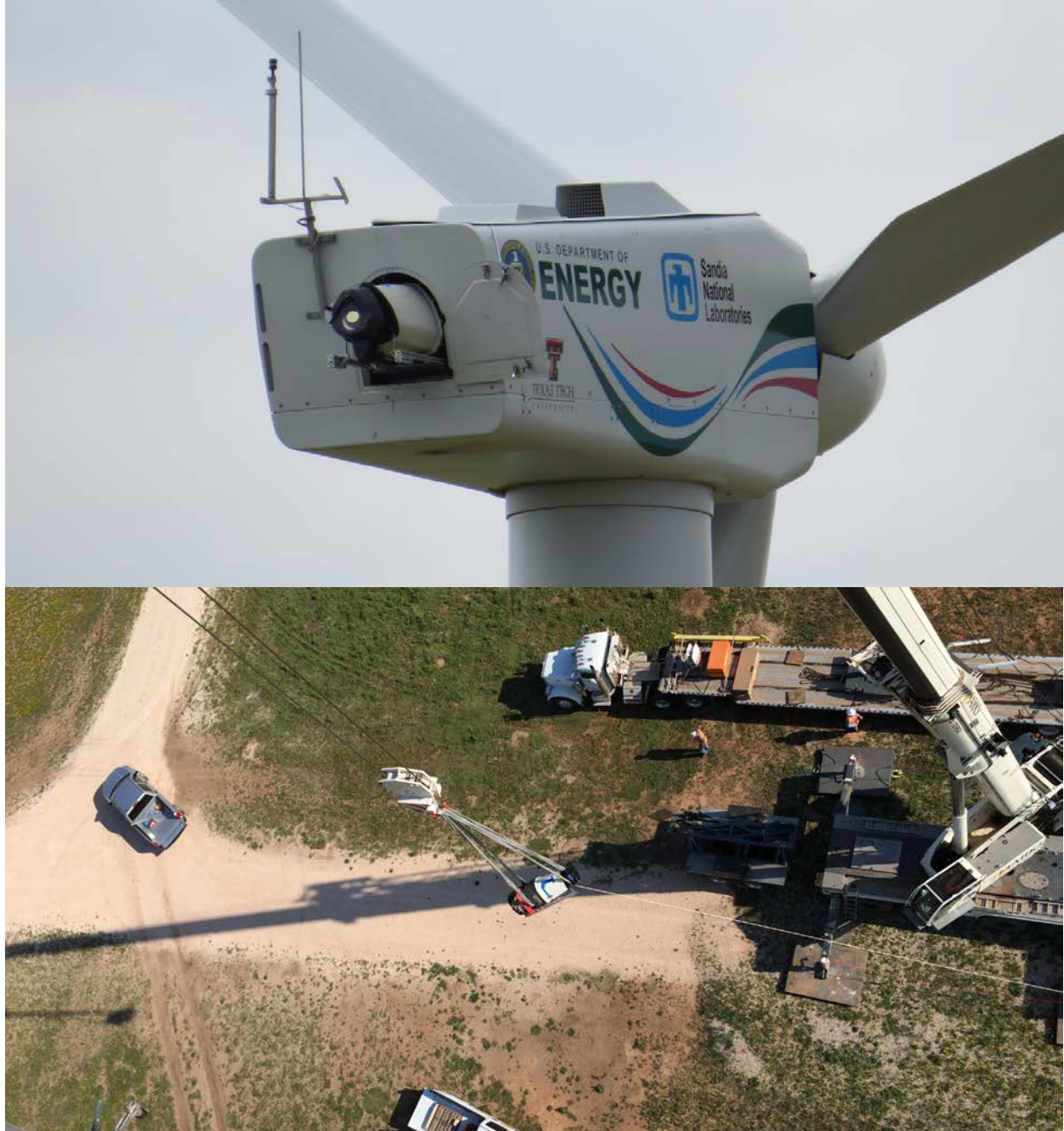
Figure 35. The SpinnerLidar fully installed in the turbine (top) a view from the nacelle of the SpinnerLidar being lifted (bottom).
