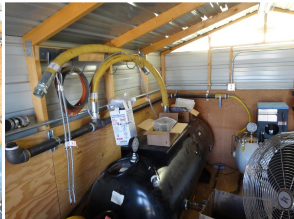
Figure 55. 240 gallon air receiver with auto drain and pressure relief valve
