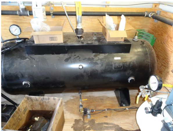
Figure 55. 240 gallon air receiver with auto drain and pressure relief valve
