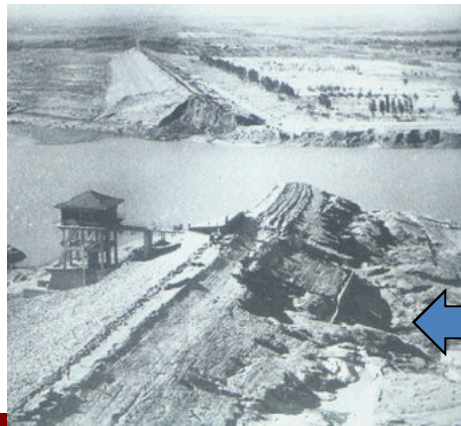
Banquiao and Shimatan Reservoir Dams (1975): structural failure 50K – 150K deaths
