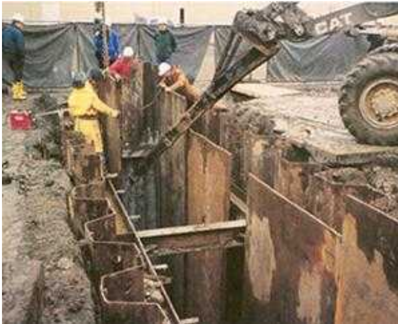
Trenching Followed by Backfilling with a Reactive Media
