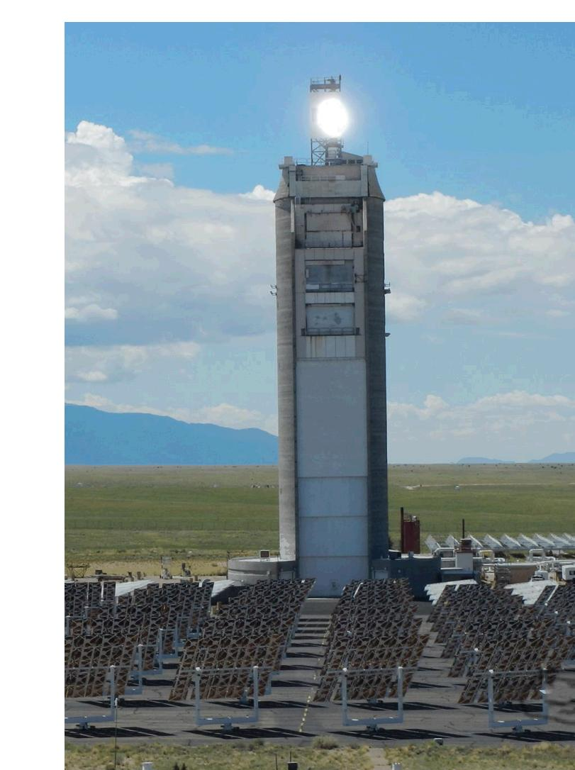
1 MW<sub>t</sub> falling particle receiver provides >720 °C particles to heat exchanger
