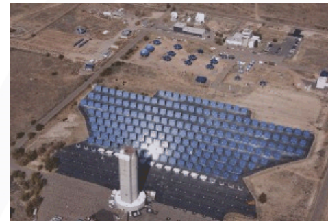
National Solar Thermal Test Facility at Sandia National Laboratories, Albuquerque, NM
