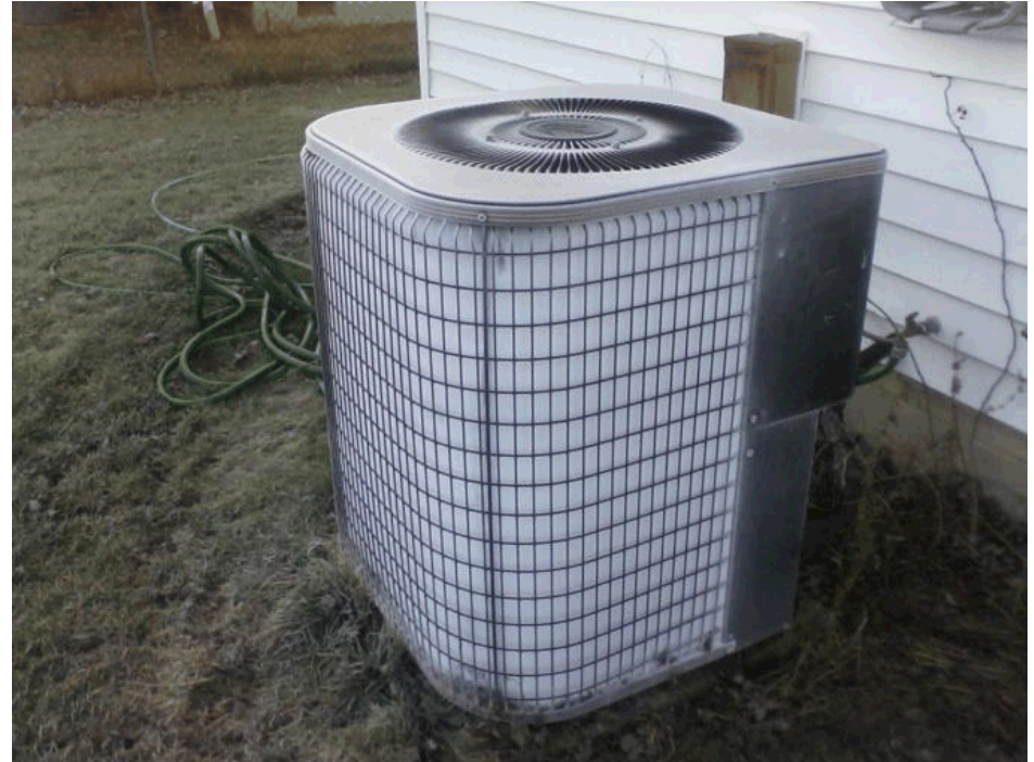
Frosted evaporator in cold climates 5
