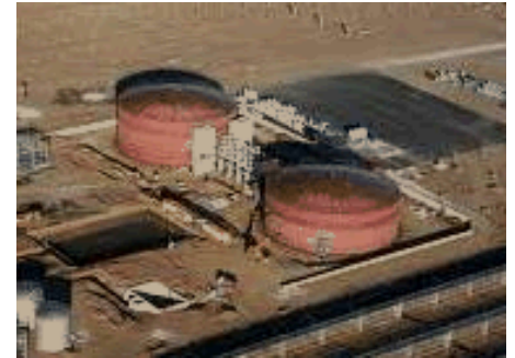
Molten-salt storage tanks at Andasol parabolic trough plant in Spain
