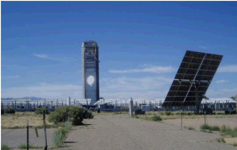
Mirror canting and gravity sag can affect optics (J.Yuan)
