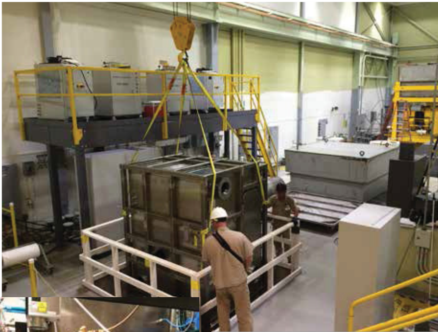
The welding cubicle, enabling development and testing of advanced welding techniques on irradiated materials, is lowered into the hot cell. The friction stir weld system (inset photo) was successfully tested.
