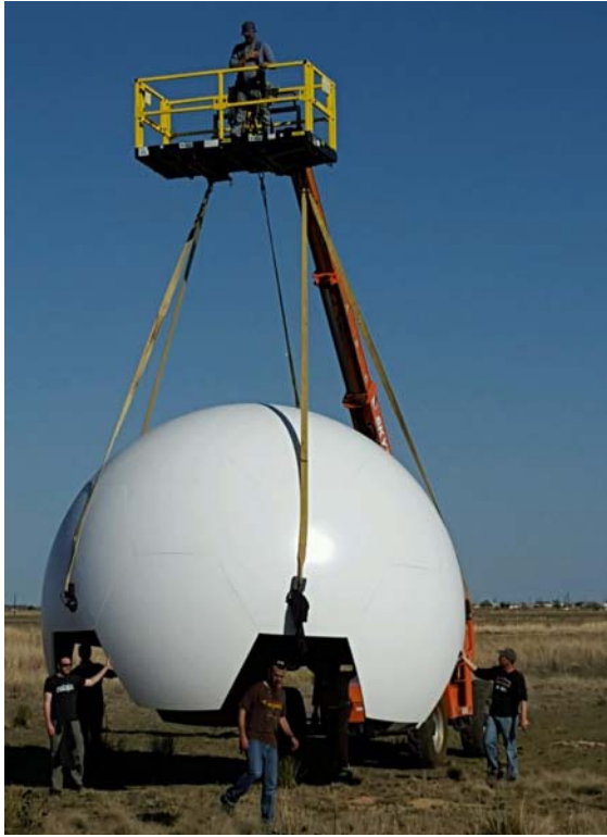
Figure 14. Upper section of radome being moved to the site.
