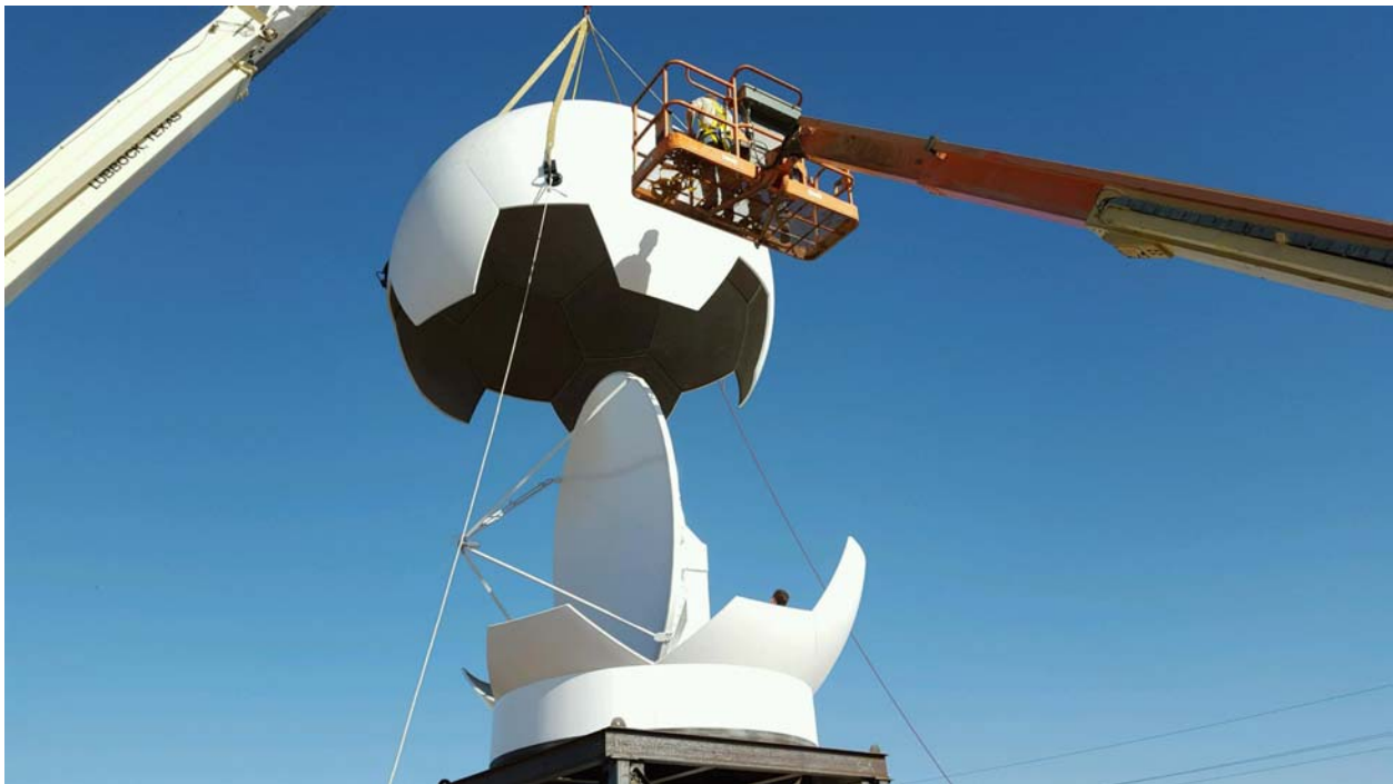
Figure 15. Upper portion of the radome being lifted into place.
