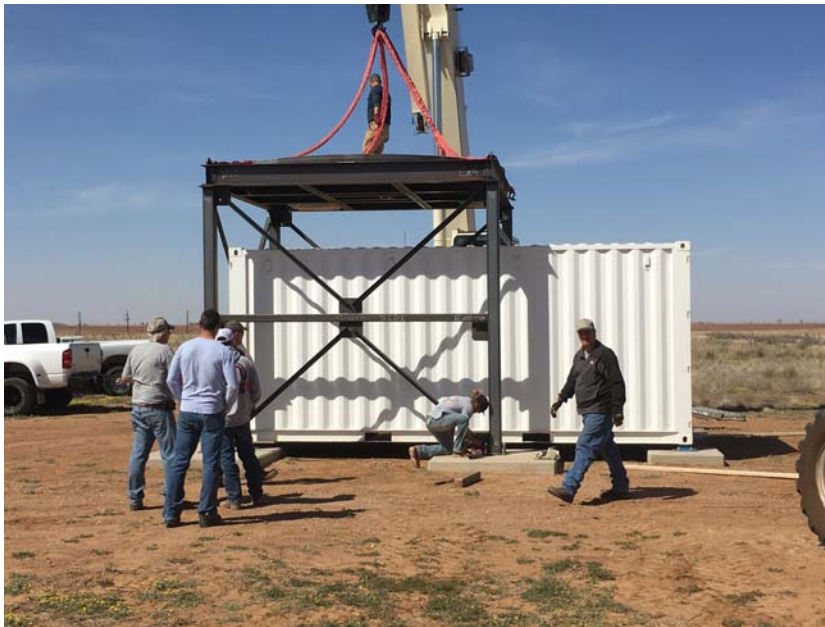
Figure 13. Phase one of the radar prototype installation at the site, as the sea container and exoskeleton platforms are mounted to the foundation.
